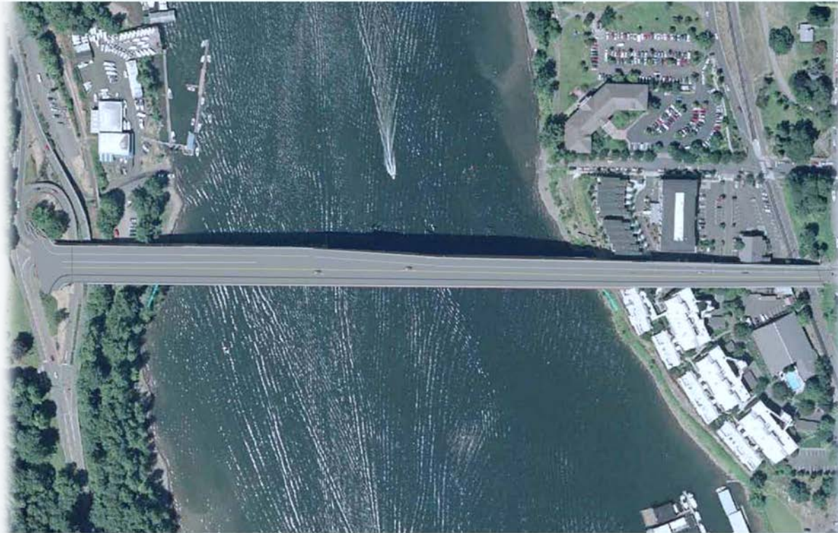
Finished Bridge, Options 1 and 2
