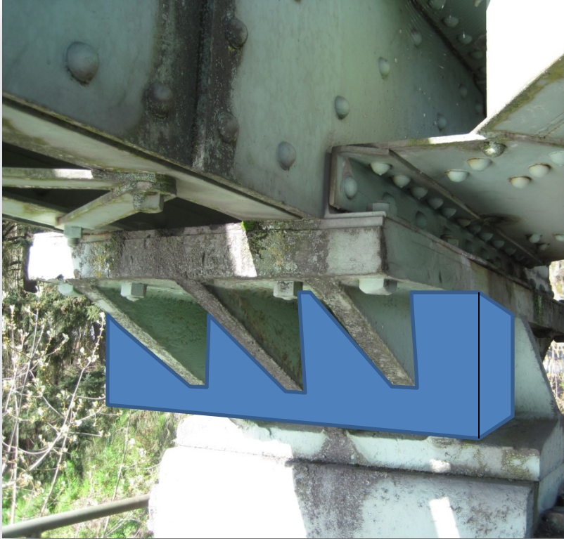
Sides cut to fit irregular shape of the bearing casting
