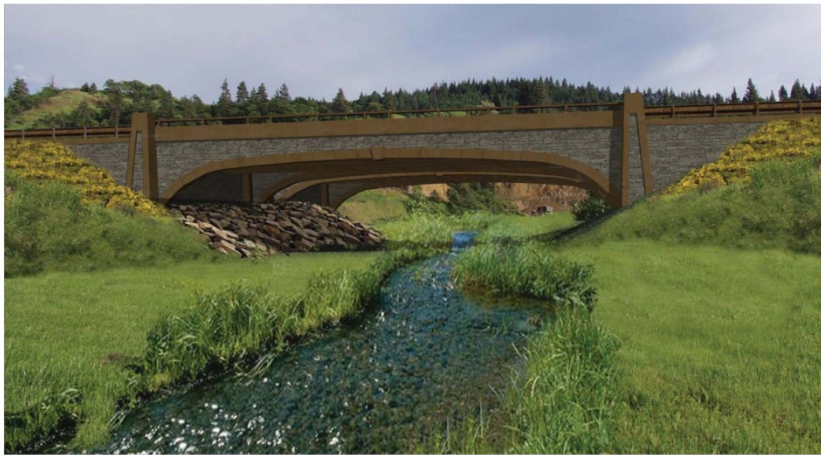
Cascadian single-span mainline bridge
