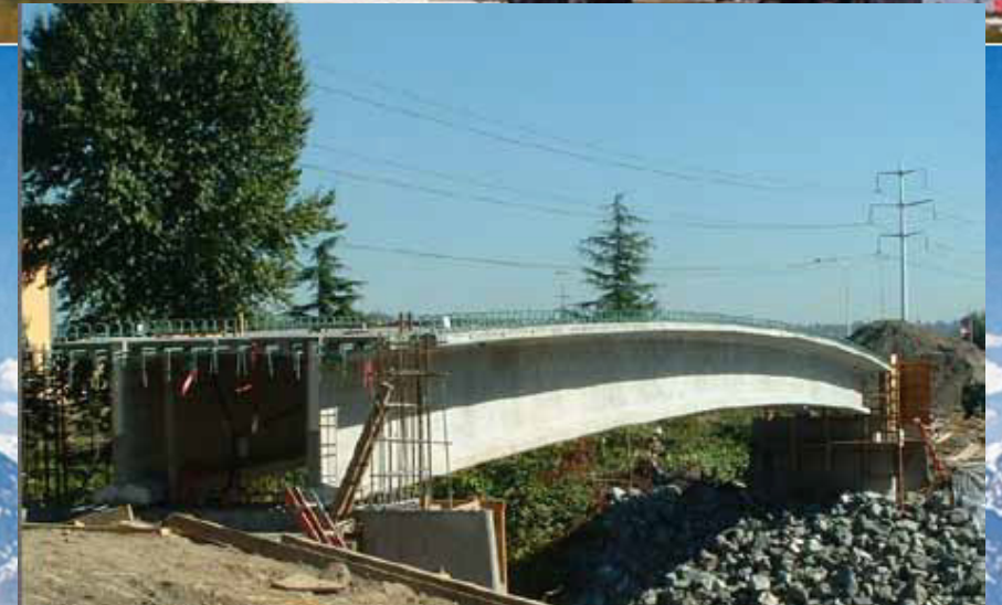
Substantially higher curvatures can be achieved using formwork
