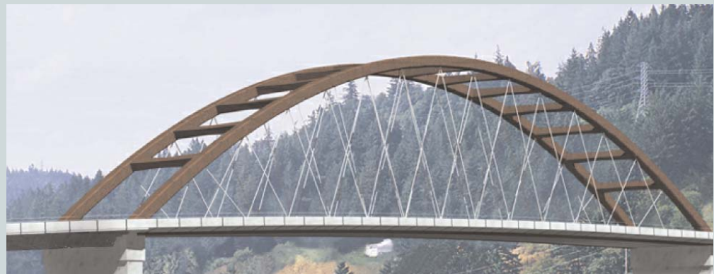
Cross cables (network)
