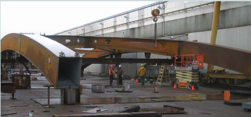
Arch ribs and top lateral bracing
