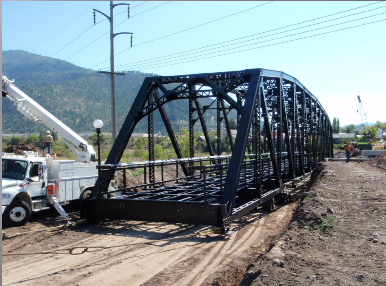
Main Span (From Behind)
