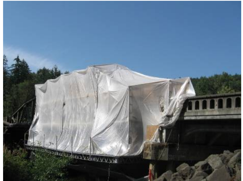
US 12 Black River Bridge No. 12/76
