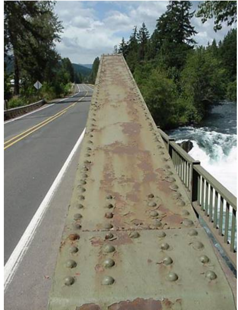
SR 141 White Salmon River Bridge (21 years)
