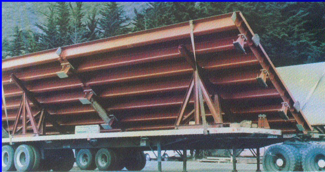
— Finished deck panel — shipment to site.
