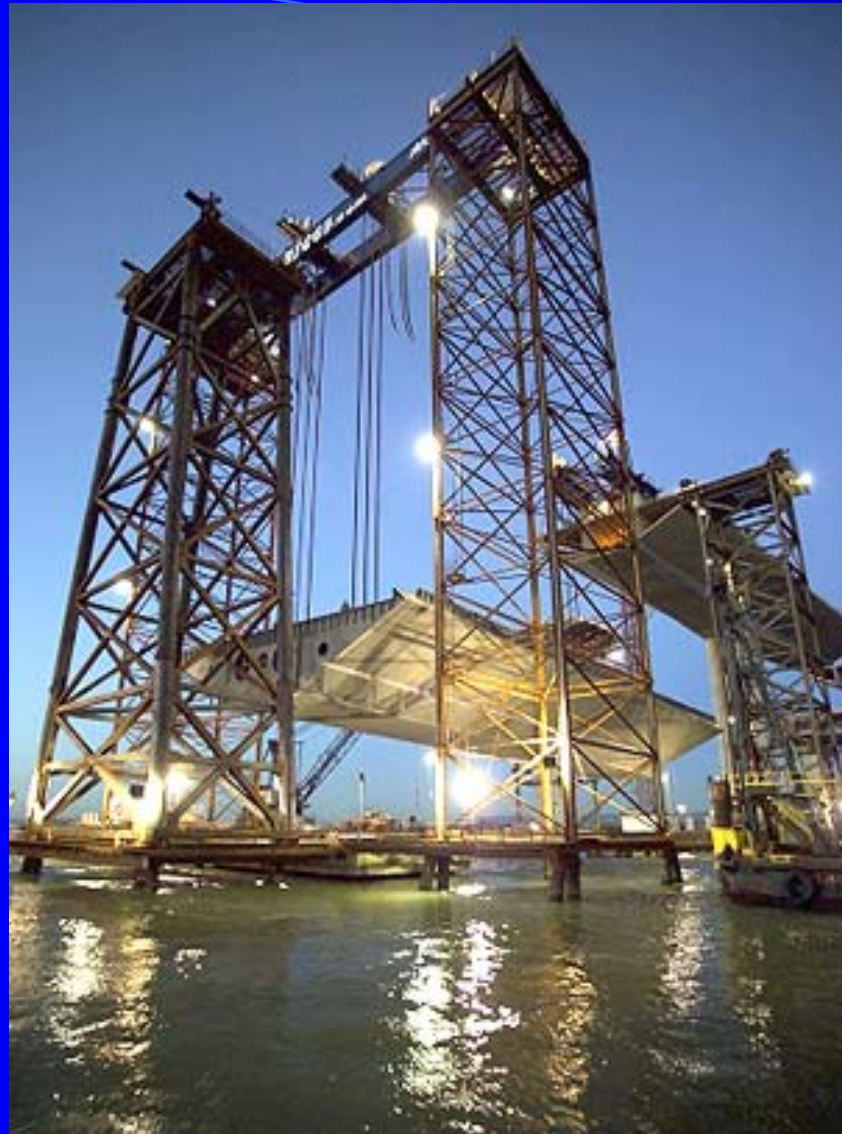
Lift of Skyway Orthotropic Spans – Fabricated by Universal Structures Inc and Oregon Steel
