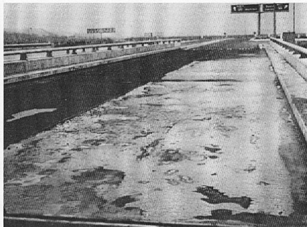
REMOVAL OF FAILED WEARING SURFACE MATERIAL
