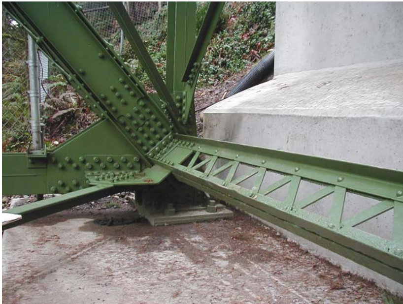
Hinged Bearing Support at East End of Bridge
