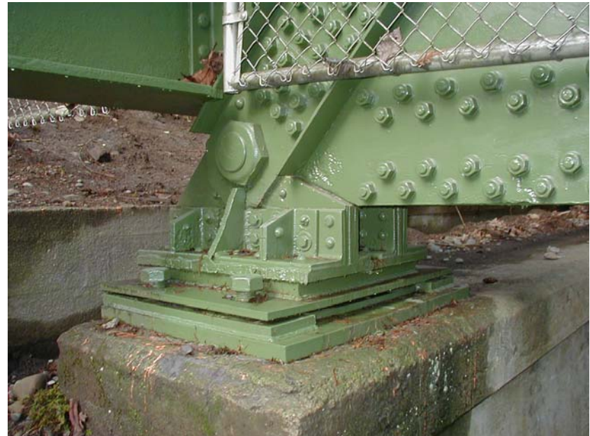
Sliding bearing support at West End of Bridge
