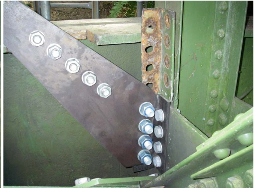
New Connection (before painting) Plate: t=1/2 ", Grade 50 Bolt: 5-7/8 " \Phi , or 4-1 " \Phi , A325 2L4x3x3/8, Grade 50
