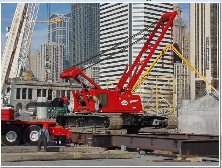
Track pressures for a large crawler crane sitting on a soft surface
