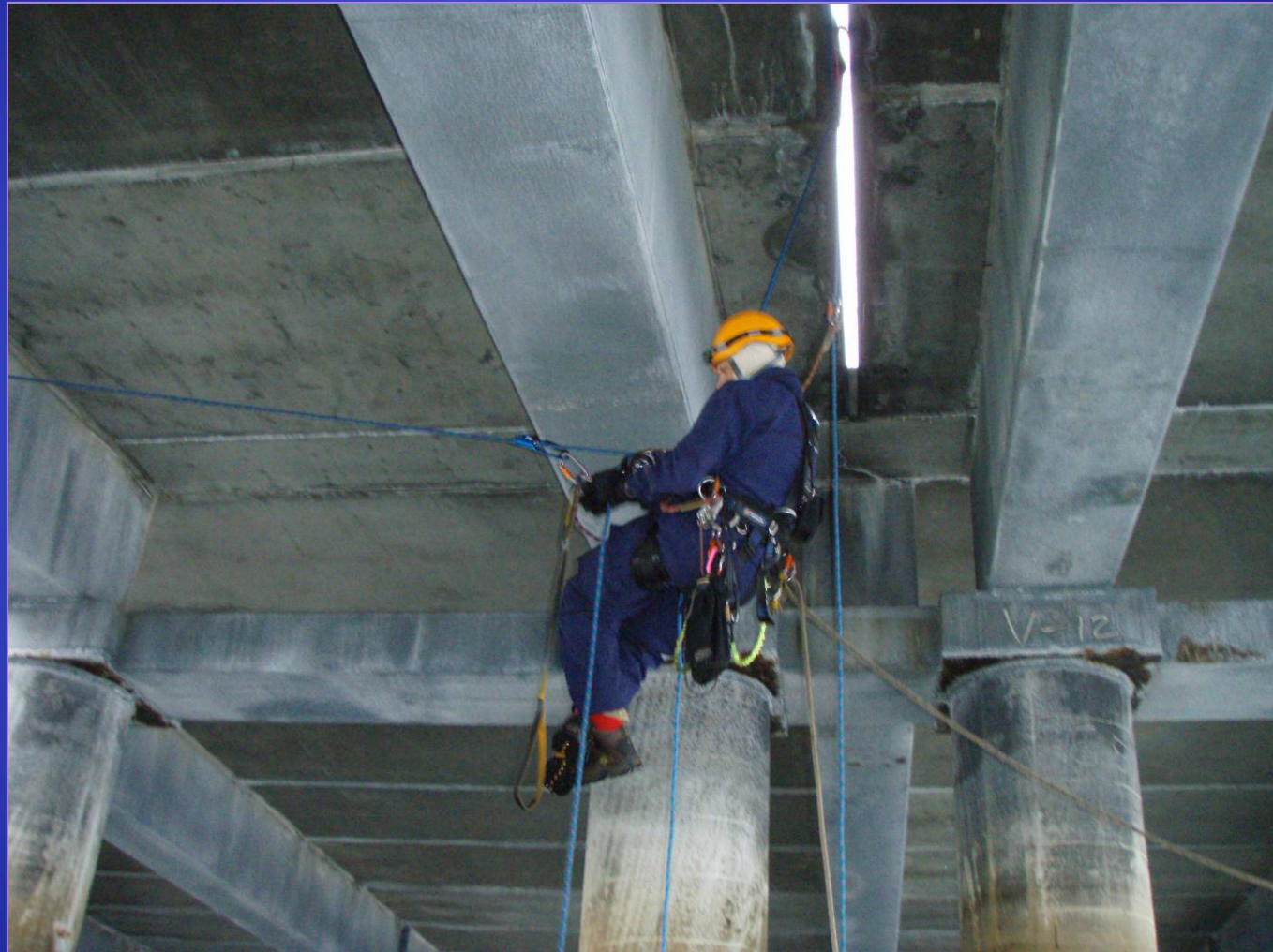
Box Girder Exterior Inspection
