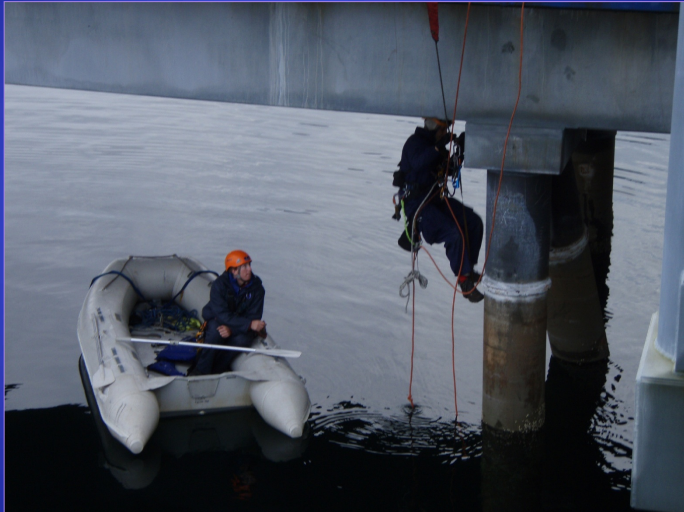
Rope Access from Boat Access
