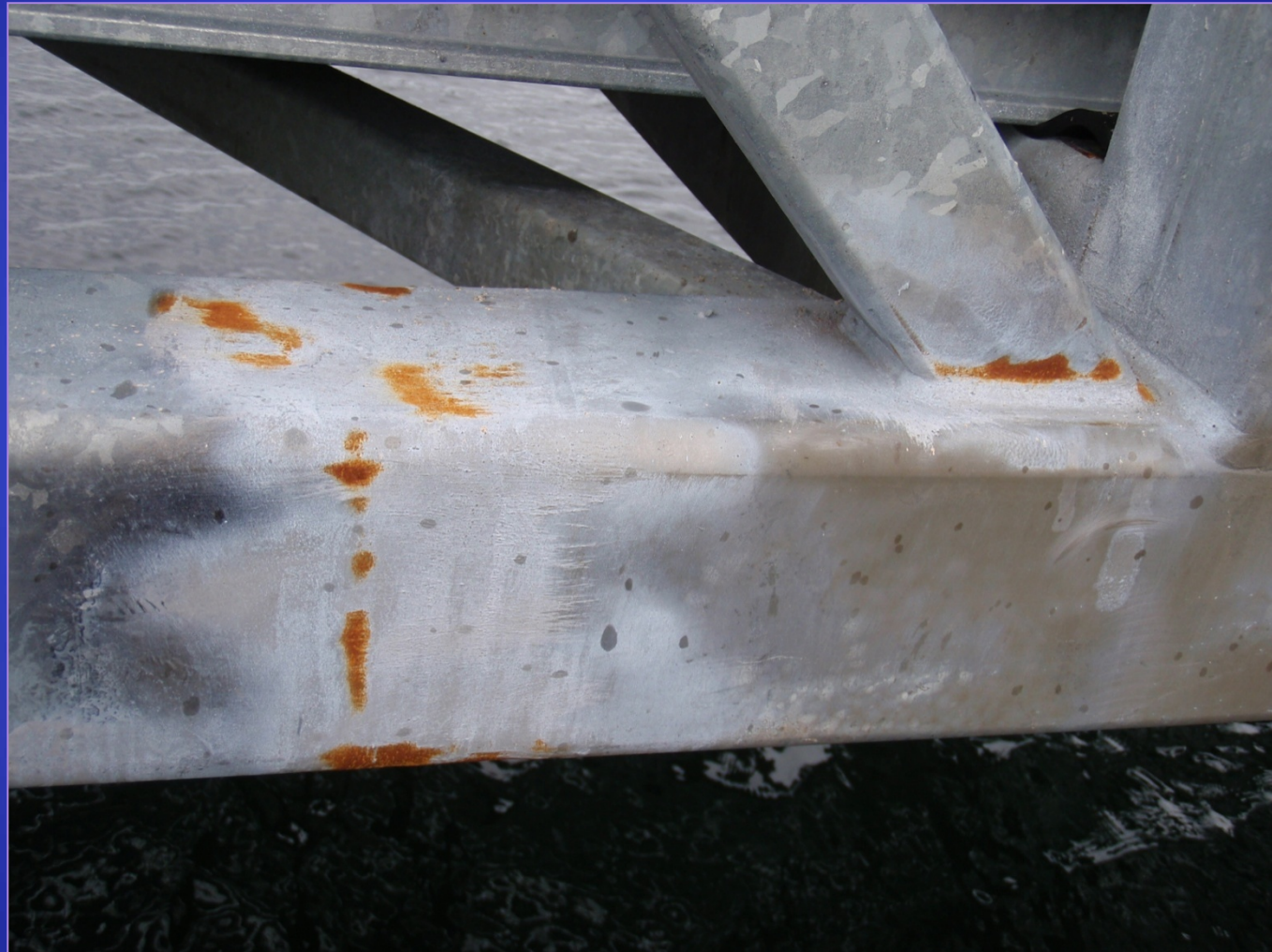
Typical Condition – Truss Members
