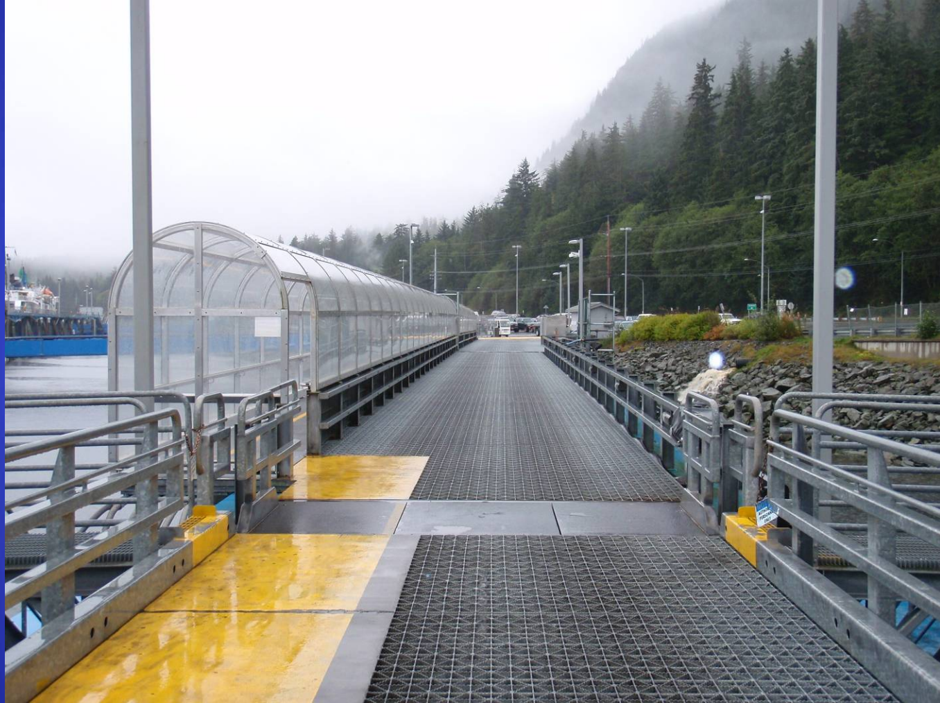
Auke Bay East Stern Berth Transfer Bridge
