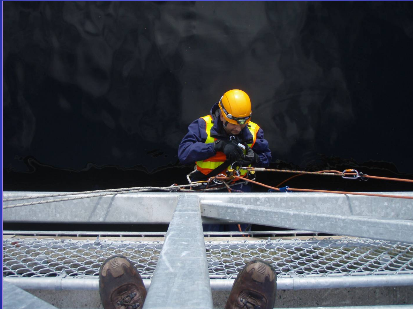
Positioned via Rope-to-Rope Transfer
