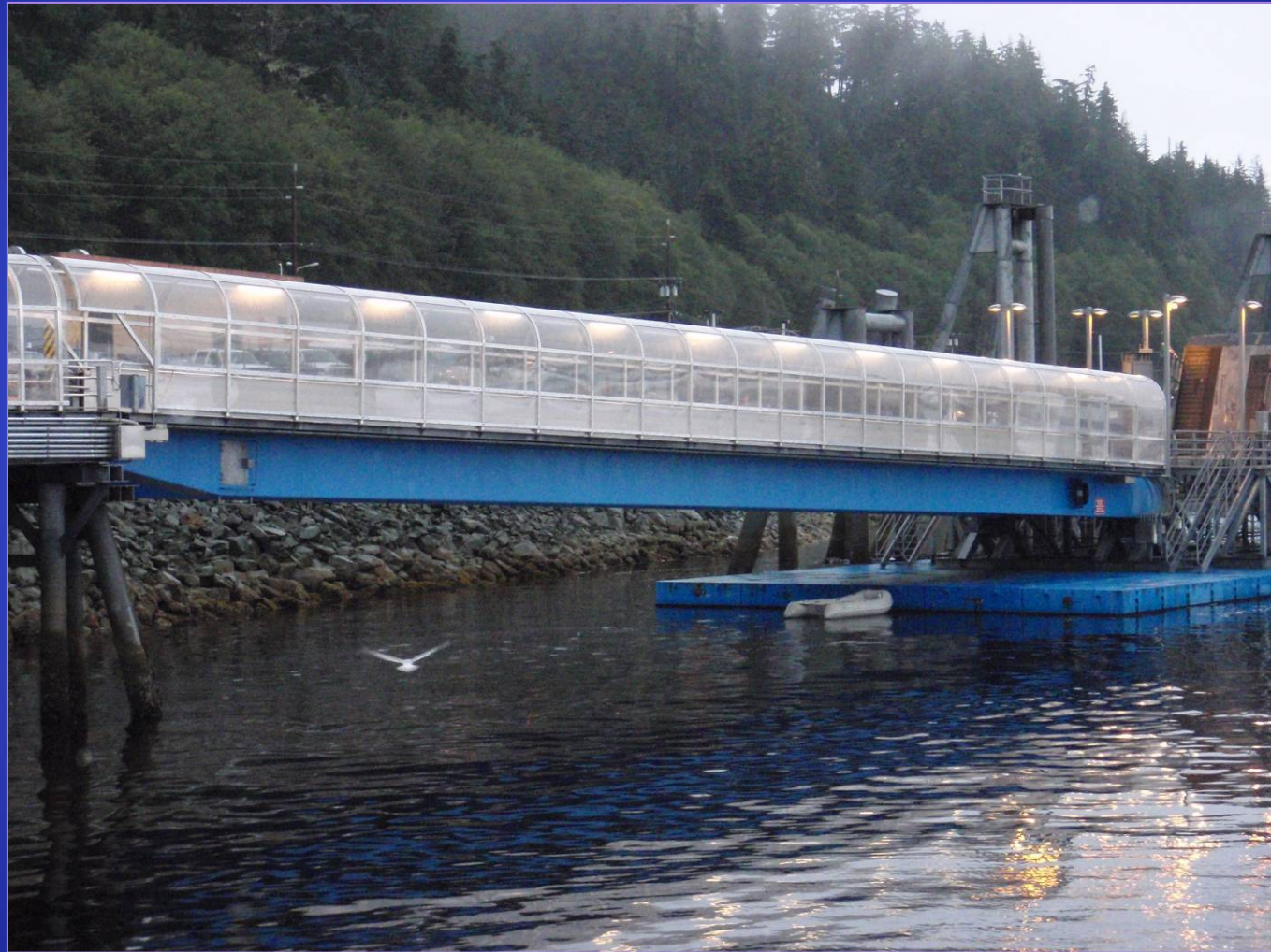
Auke Bay East Stern Berth Transfer Bridge
