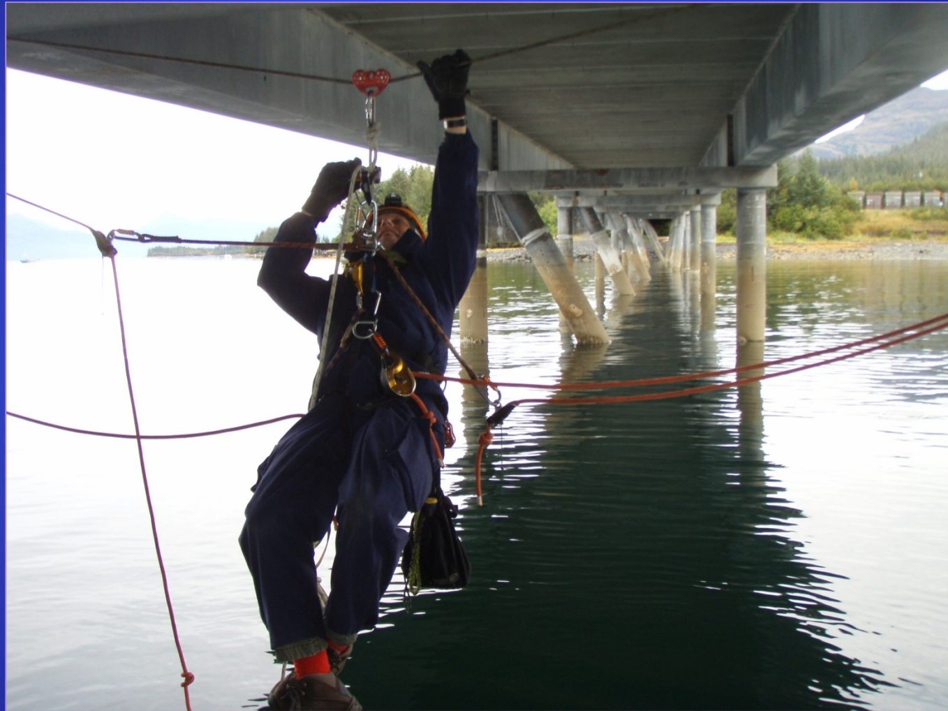
Exterior Inspection via Pulley System
