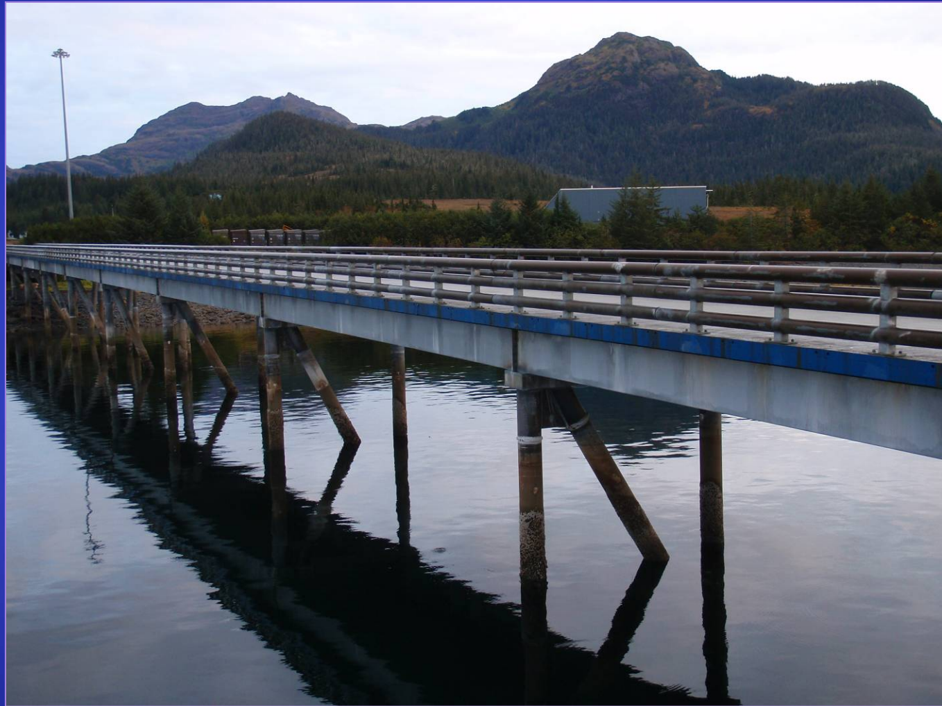
Approach Trestle Structure
