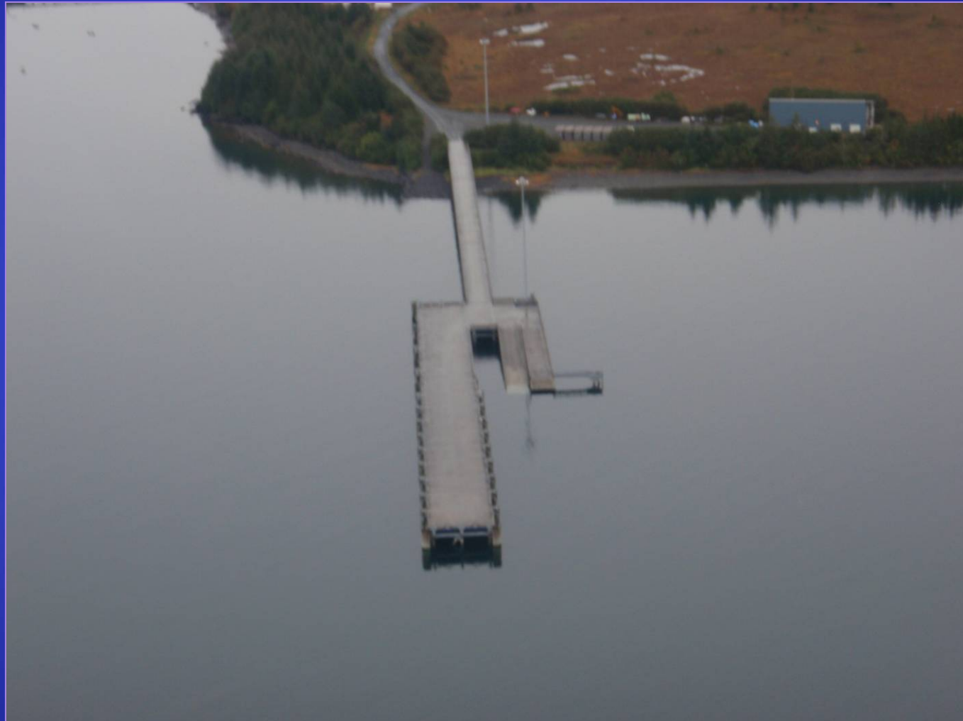
Approach Trestle, Main Dock & Tidal Ramps
