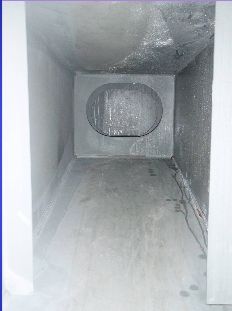
PRCS Entry - Box Girder Interior Inspection
