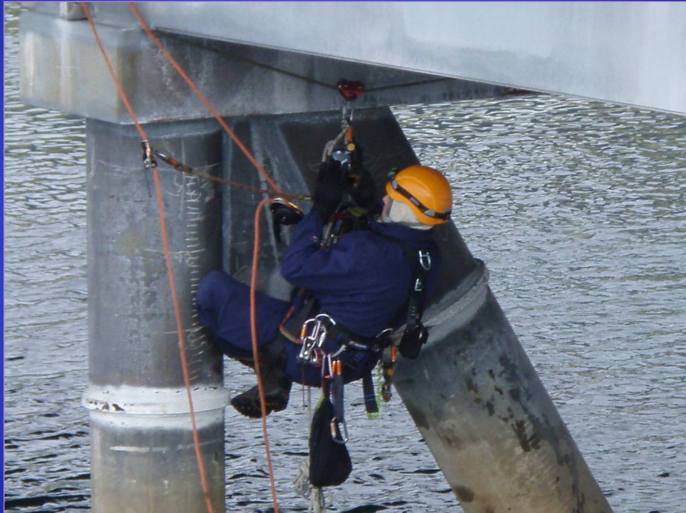
Bent Cap Exterior Inspection
