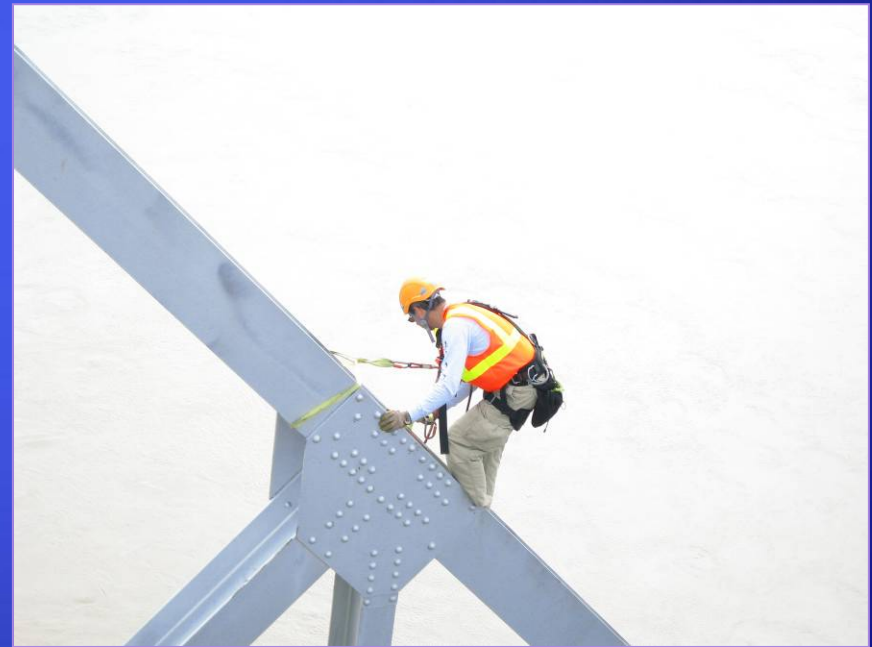
Rope Access – Structure Climbing
