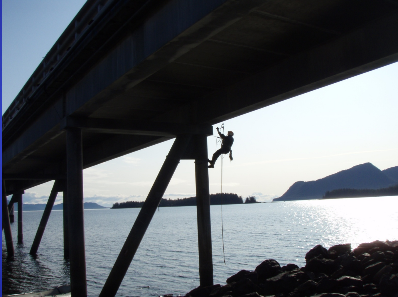
Rope Access from Ground Access
