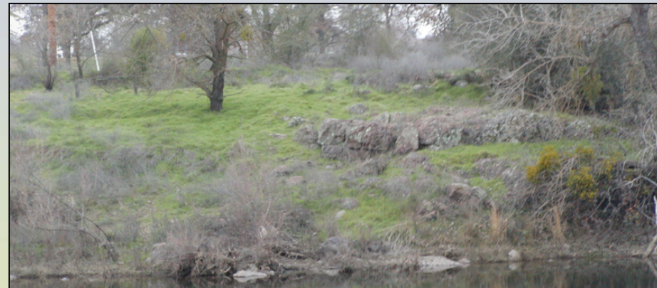
Foundations – near surface bedrock
