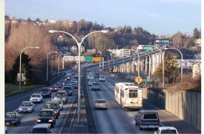
Portage Bay Bridge – Facing West
