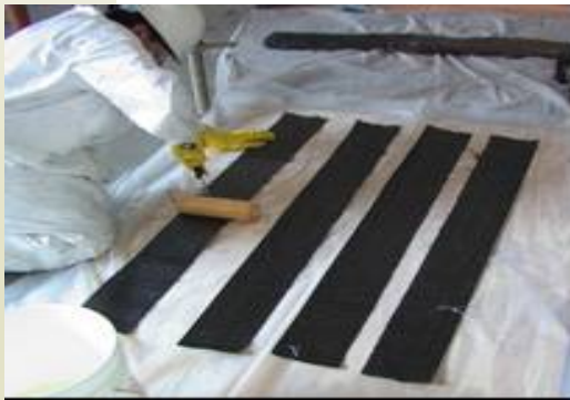
Resin impregnation of fabric
