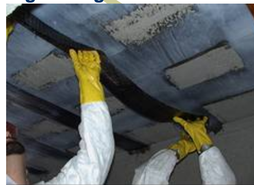
Bonding fabric to concrete
