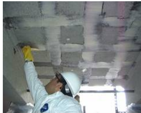
Adhesive application on concrete
