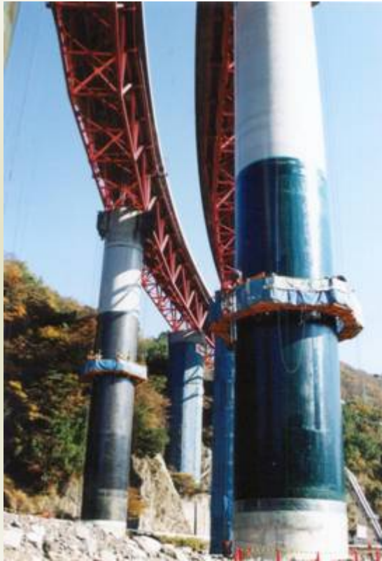
Bridge pier- confinement
