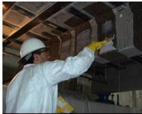
Bonding FRP to concrete
