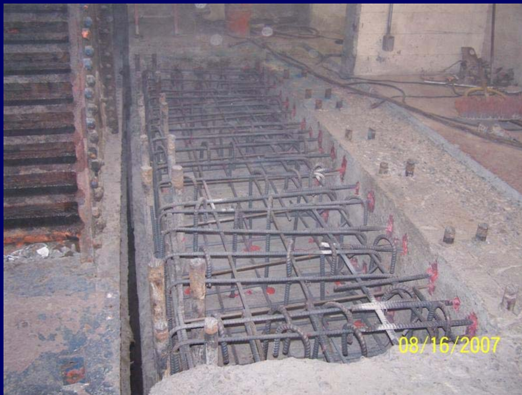
Machinery Anchorage Modifications
