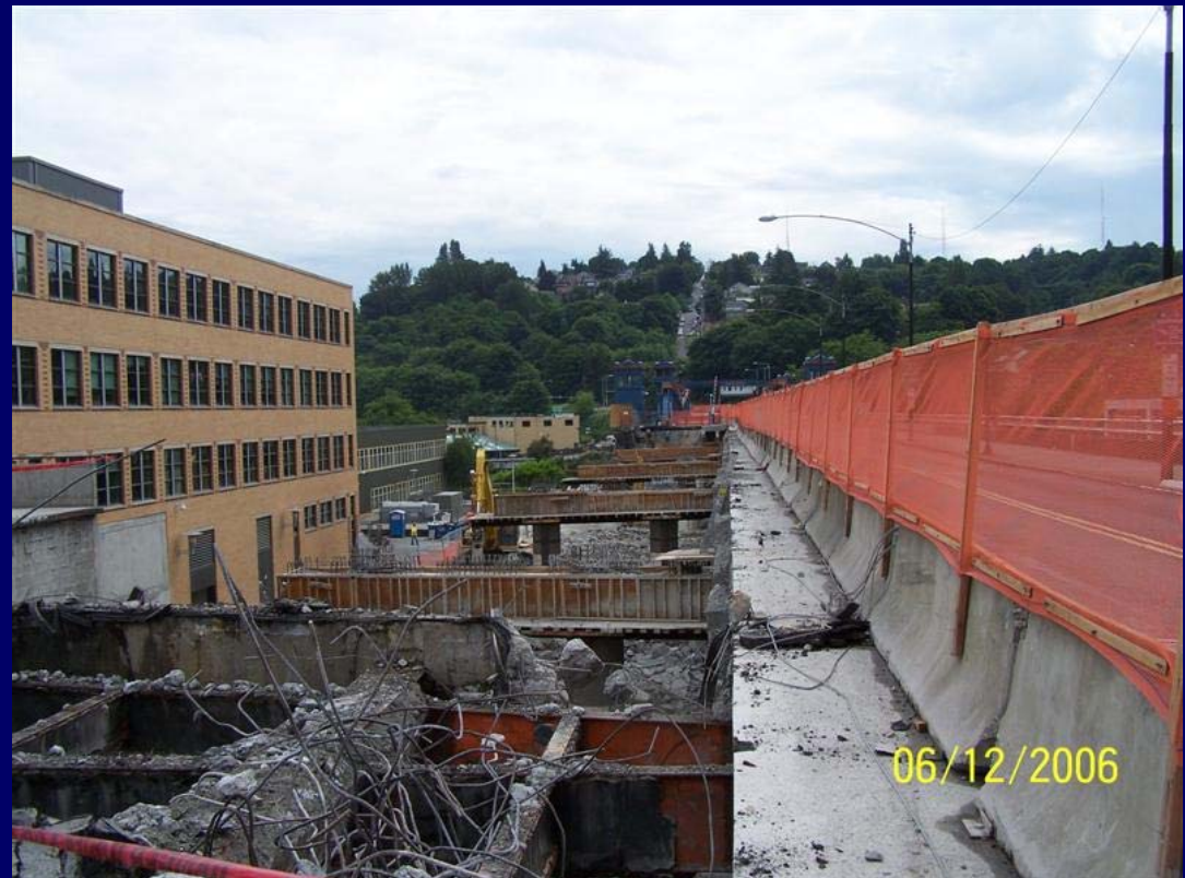
North Approach Replacement Under Construction
