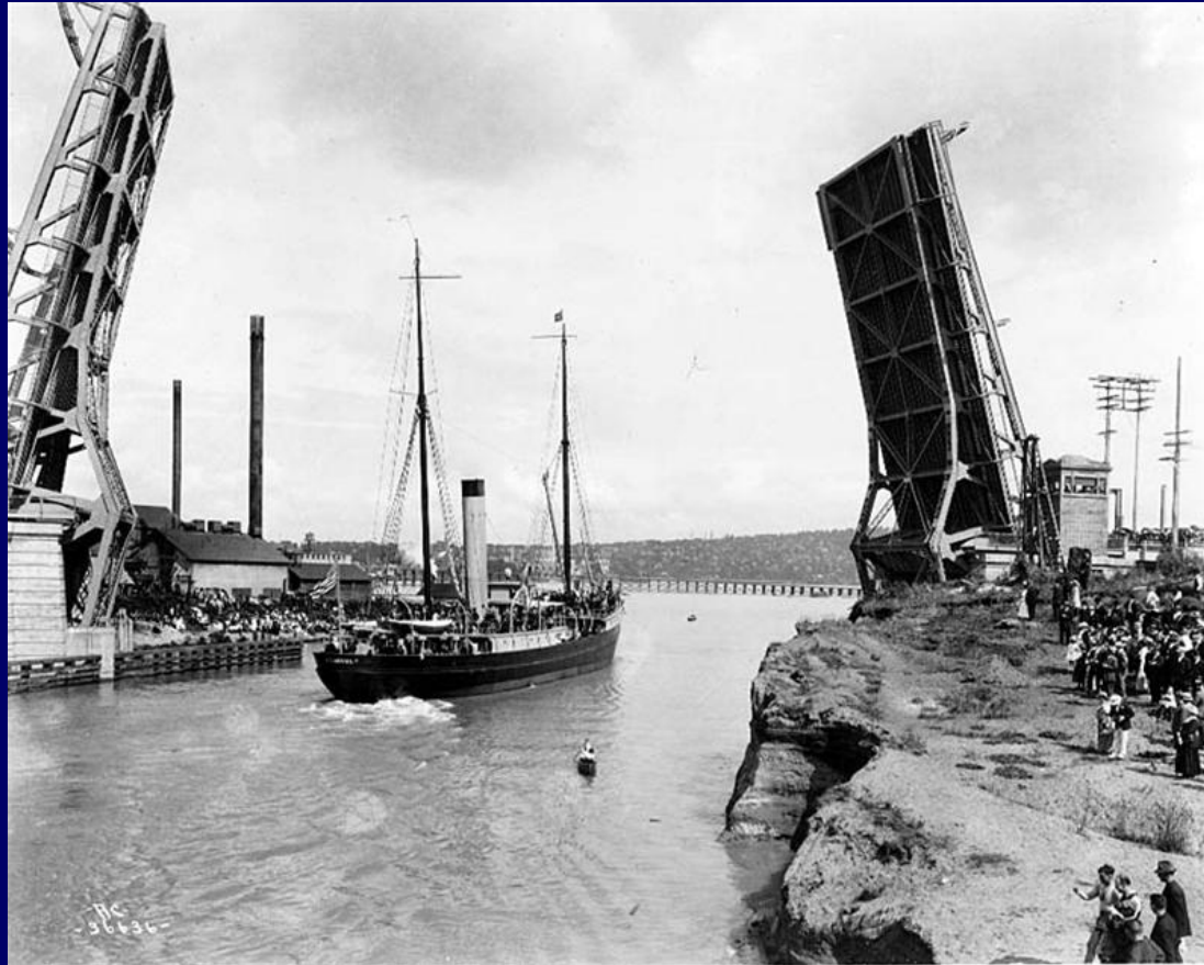
Fremont Bridge, Circa 1917 Seattle Municipal Archives Photograph Collection
