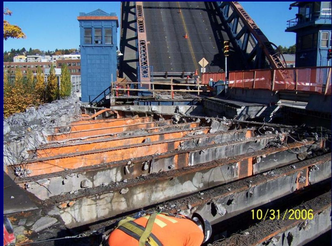
South Approach Replacement Under Construction
