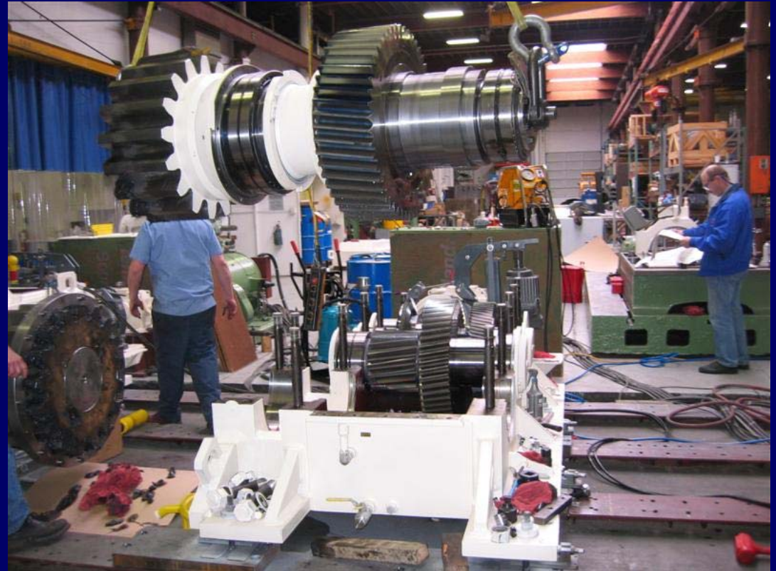
Assembly Of The Output Pinion Shaft Into The Reducer At The Gear Works, Seattle
