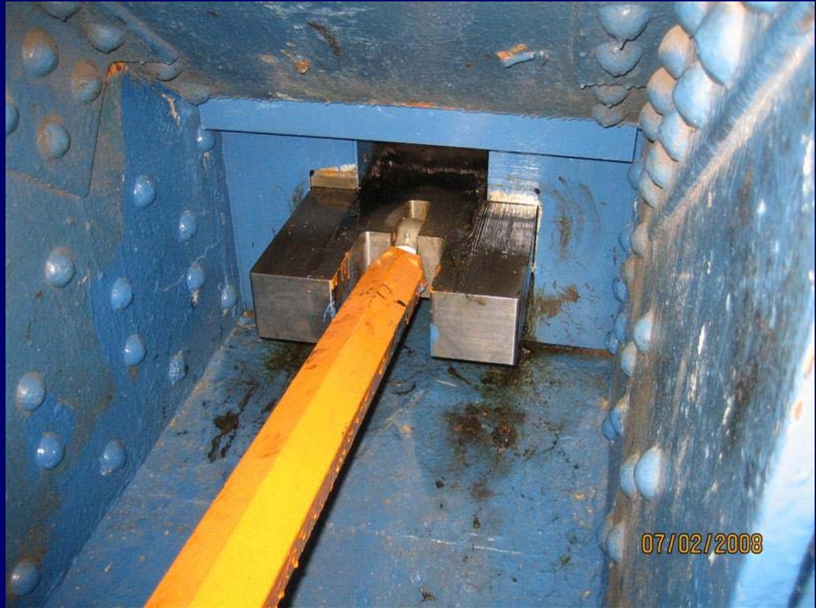
New Span Lock Connecting Rod, Lock Key And Guide With Bronze Wear Shoes, Shown Disengaged
