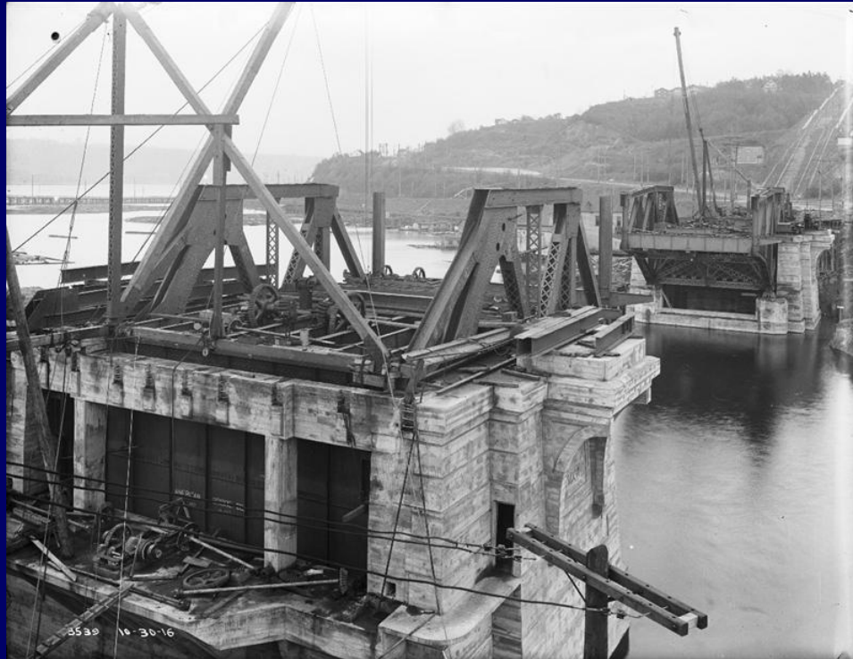
Construction of the Fremont Bridge, Circa 1916 Seattle Municipal Archives Photograph Collection
