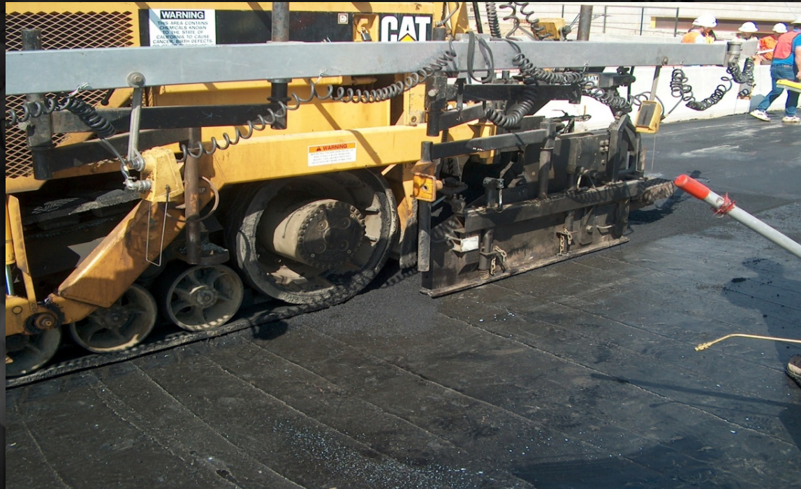
Paving over spray applied MMA waterproofing on Carquinez Bridge
