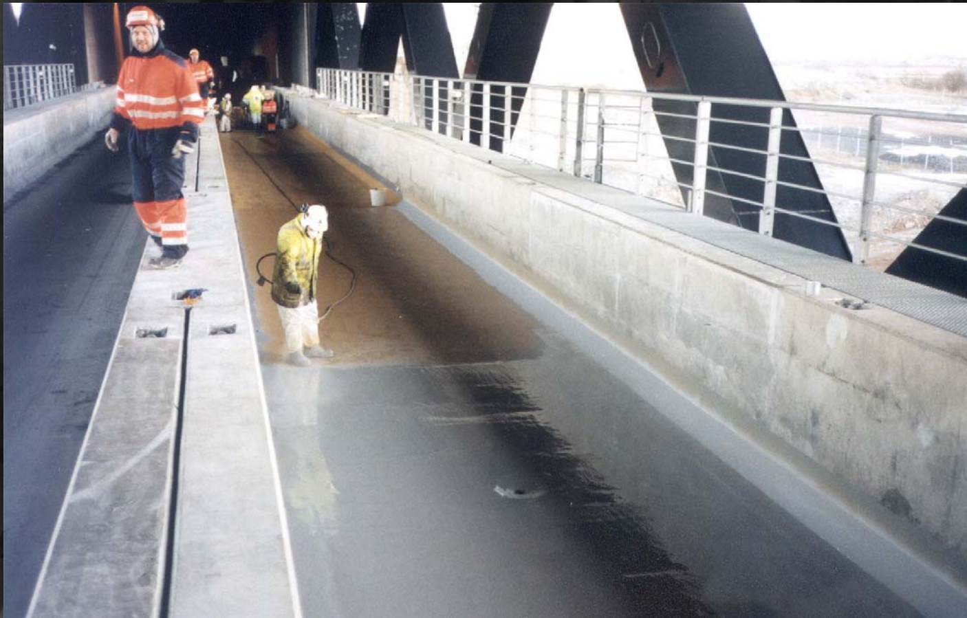
Waterproofing the Oresund Bridge between Denmark & Sweden at temperatures below freezing
