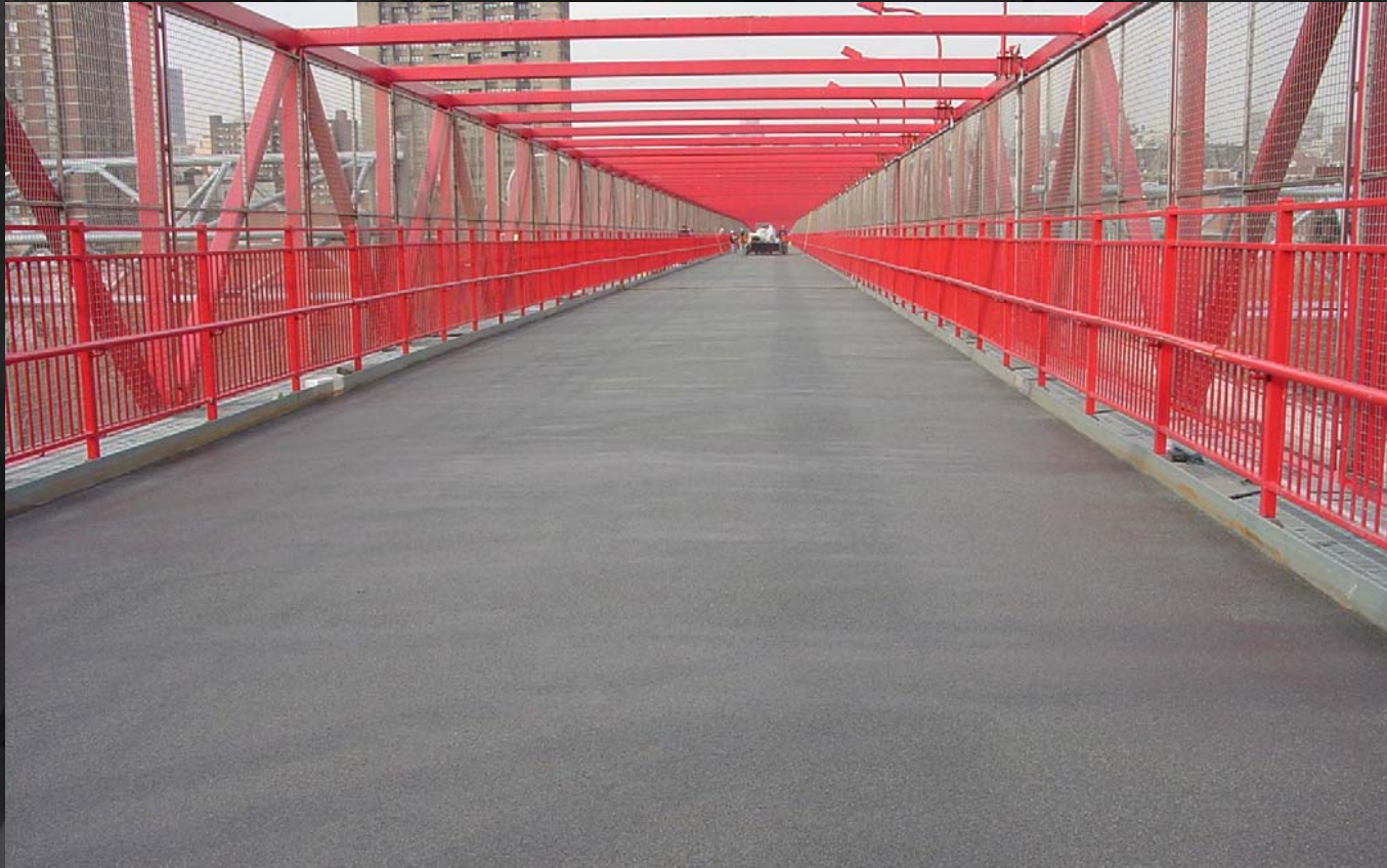
Polymer Overlay, Williamsburg Bridge, New York City
