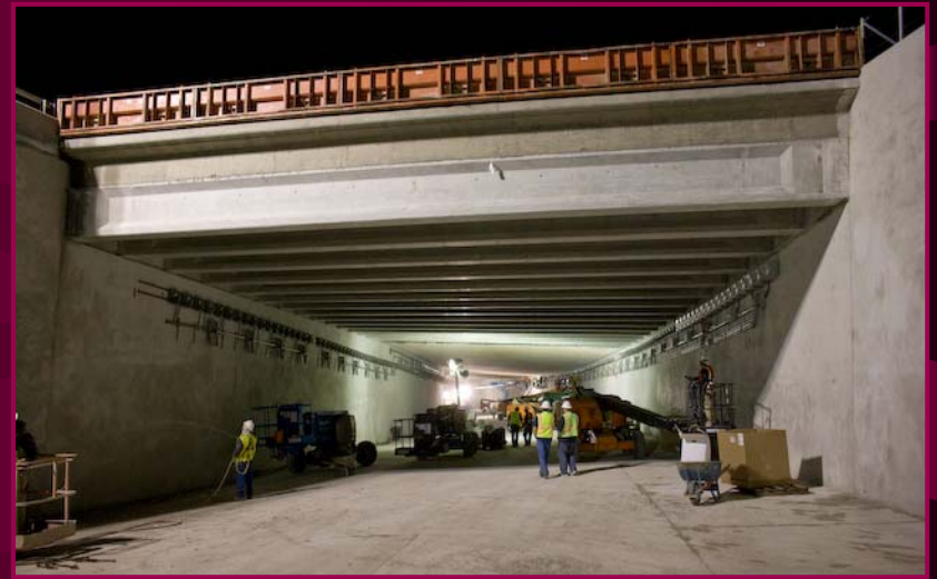
I-5 Truck Route Fire Repair - San Fernando
