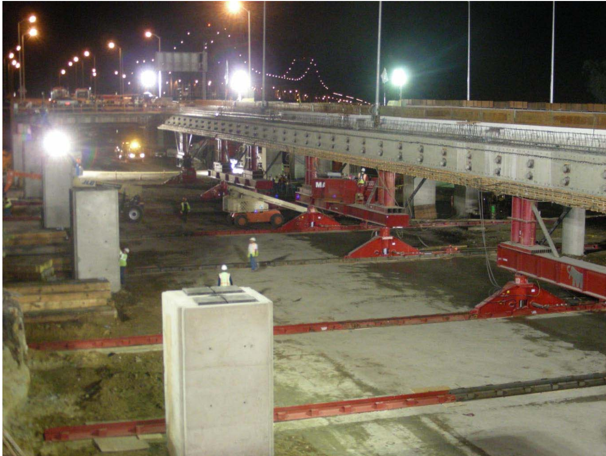
Superstructure Roll-In Move
