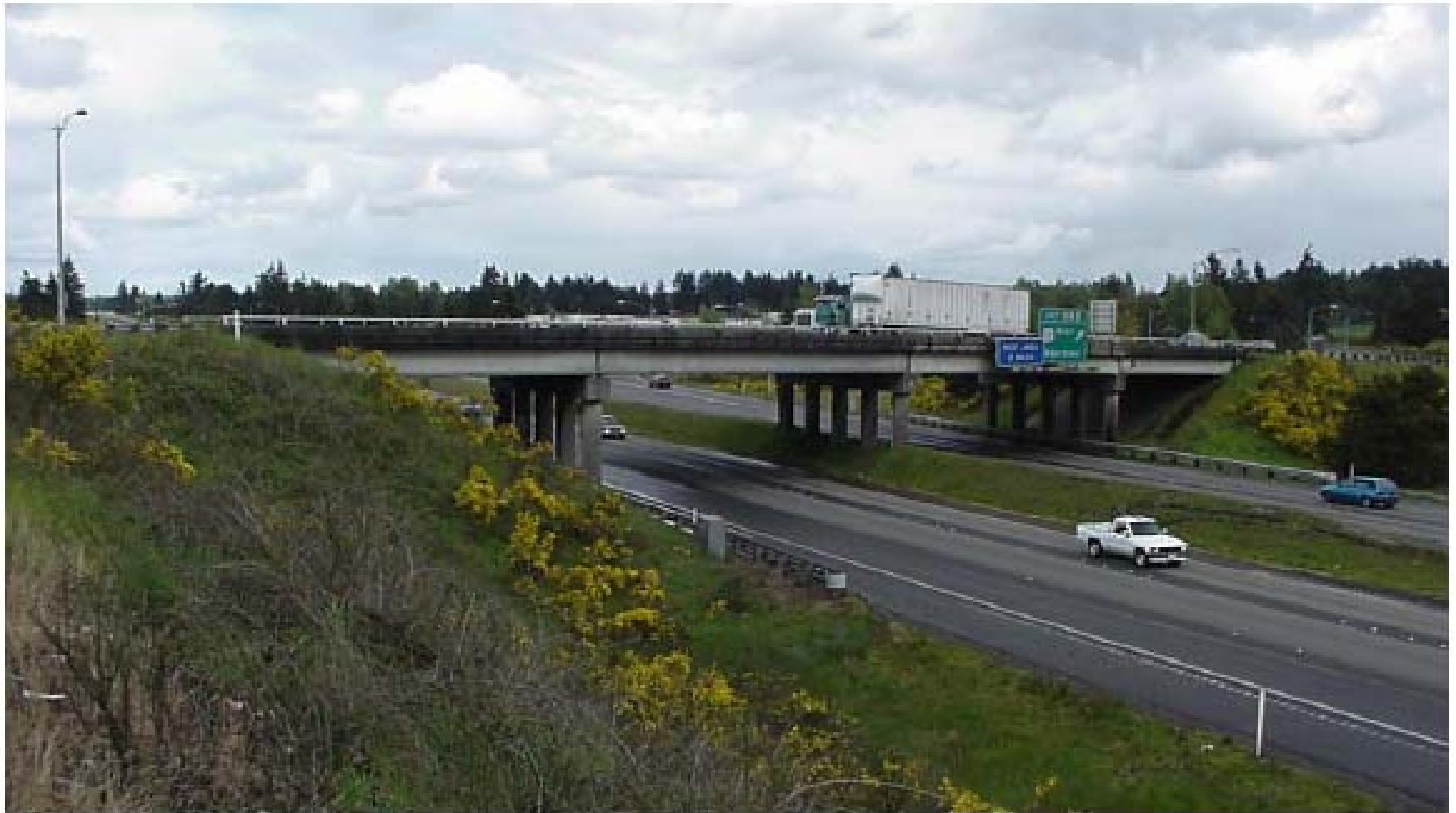
Figure 5. Existing SR 12 Overcrossing of I-5 to be Replaced
