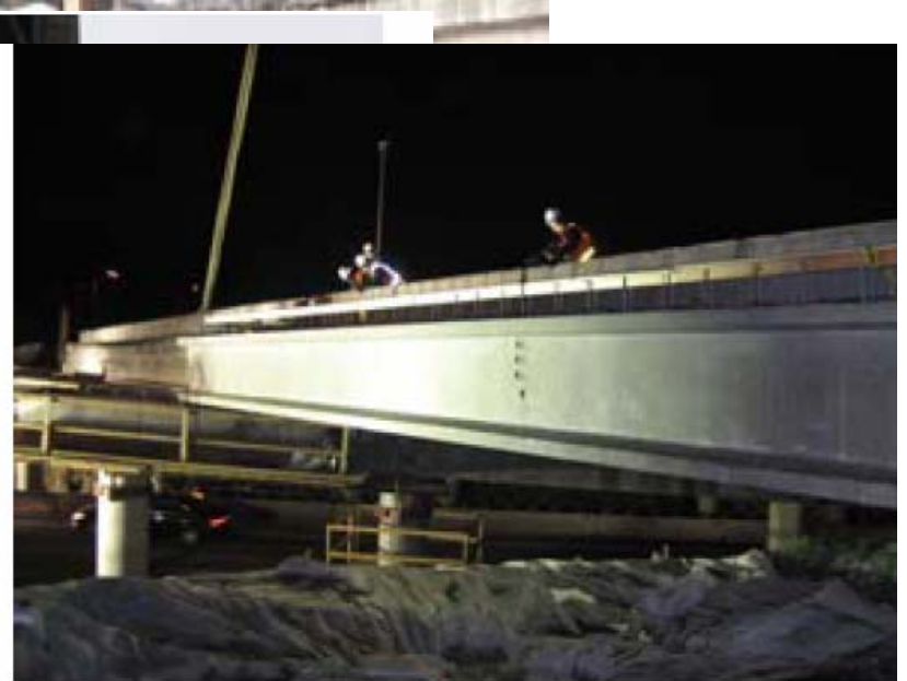
Girder set in place for the I-405 Coal Creek Parkway bridge.
