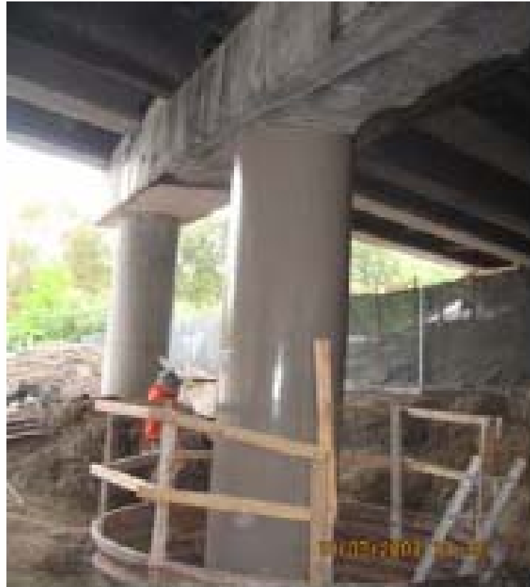
Bridge Column Seismic Retrofit at Coal Creek Parkway.
