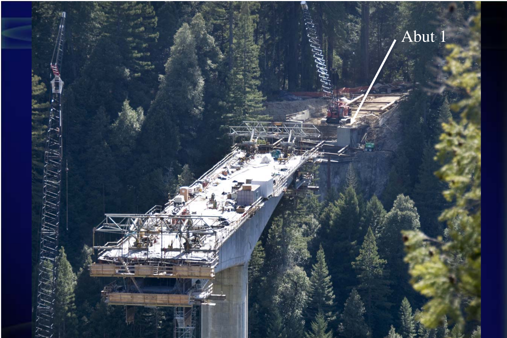
Pier 2 Cantilever construction above redwood trees
