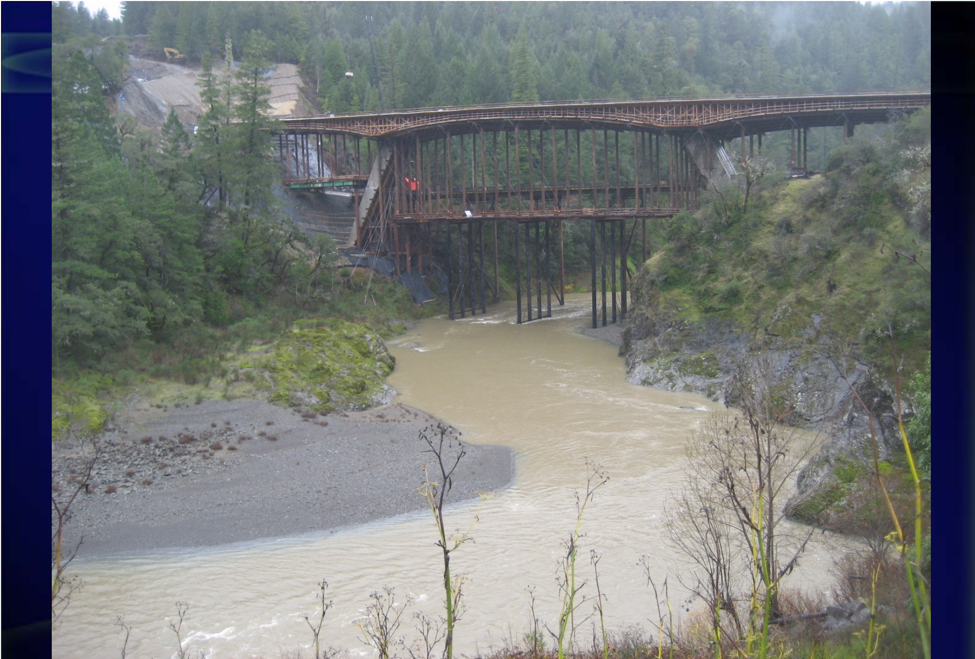
North Bridge Falsework approximately 140' tall (Temporary trestle in background)
