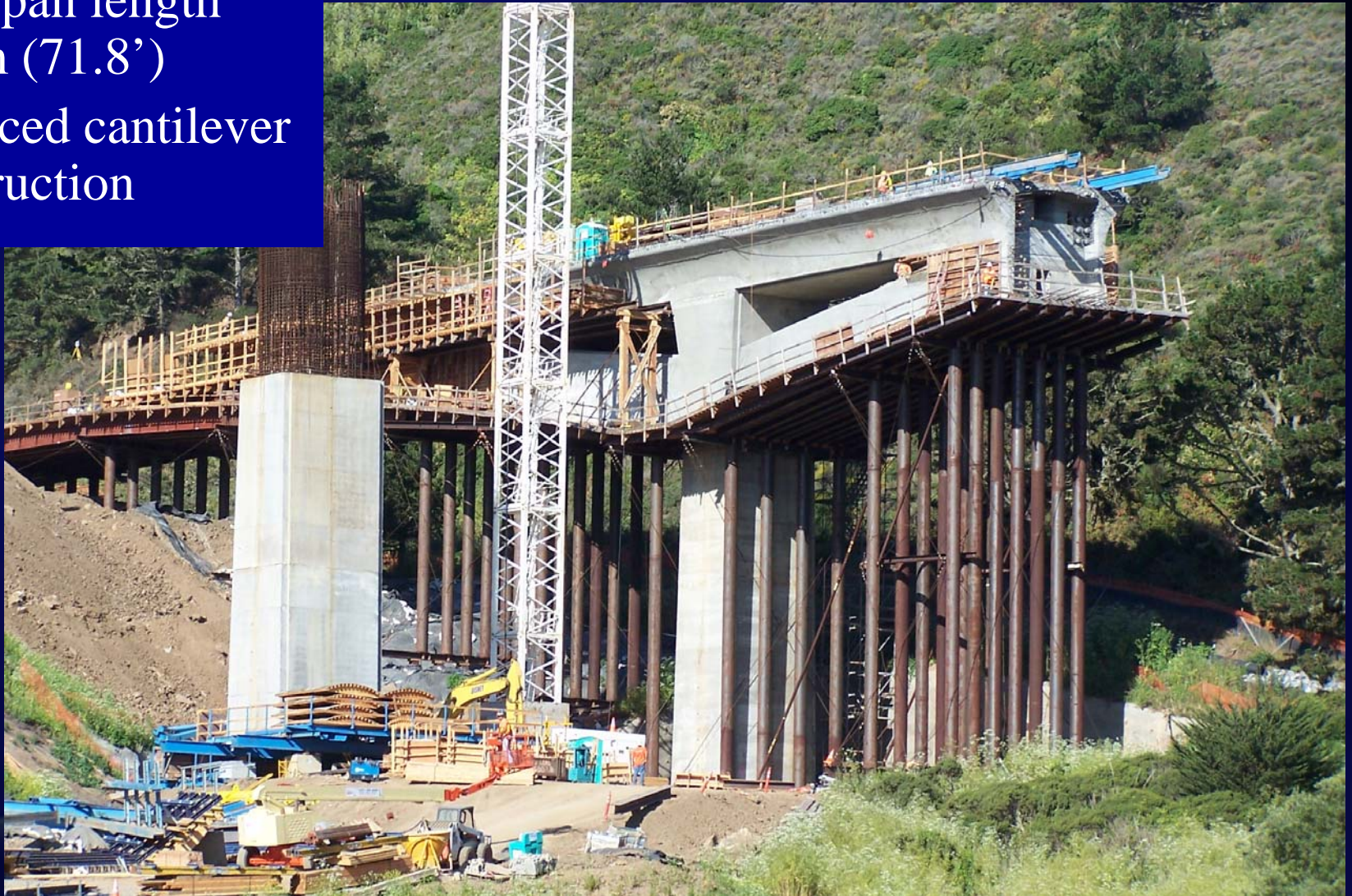
Pier Table Falsework
