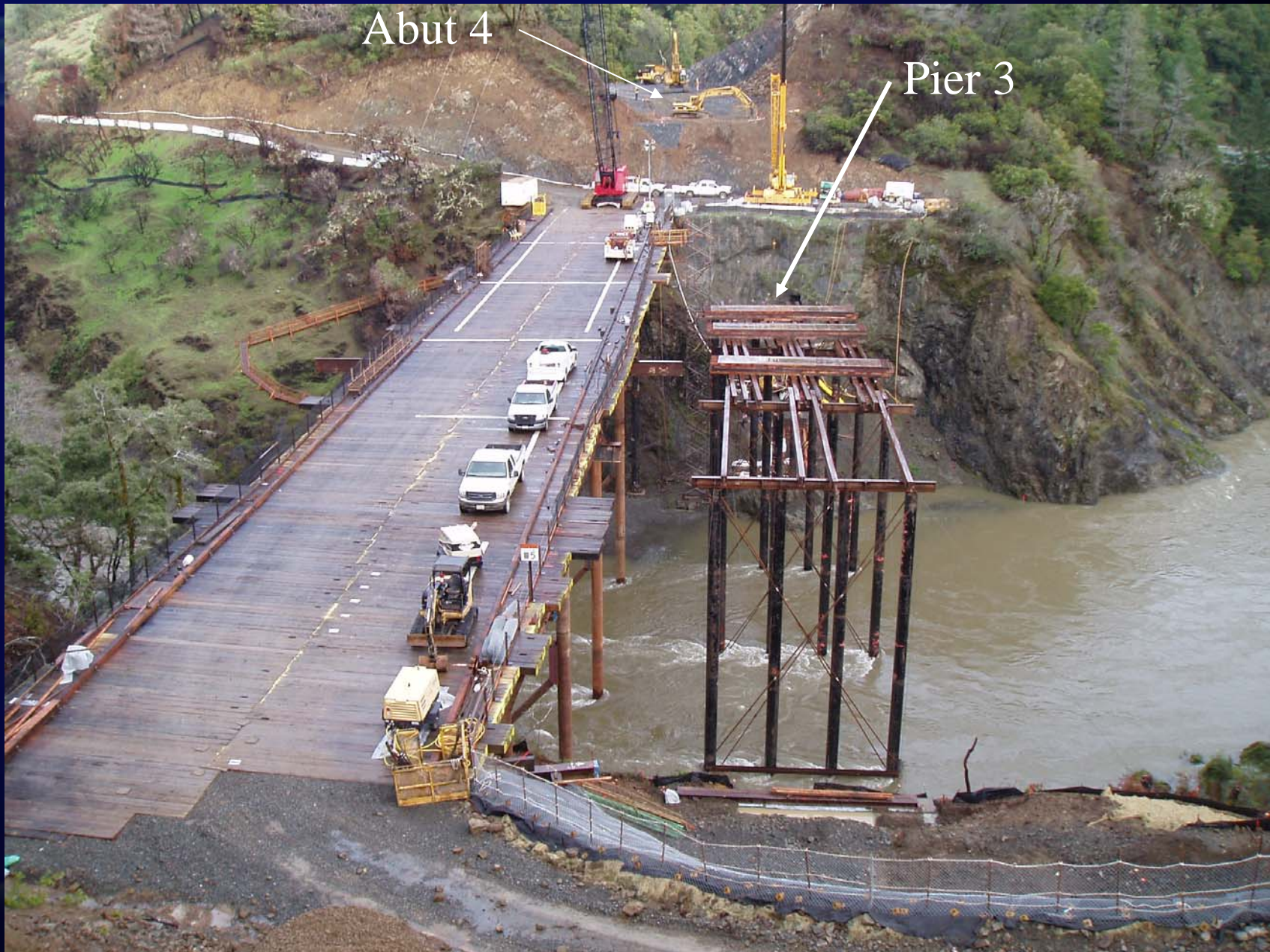
Temporary Trestle and start of North Bridge Falsework
