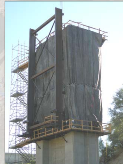
Pier Insulating Blankets
