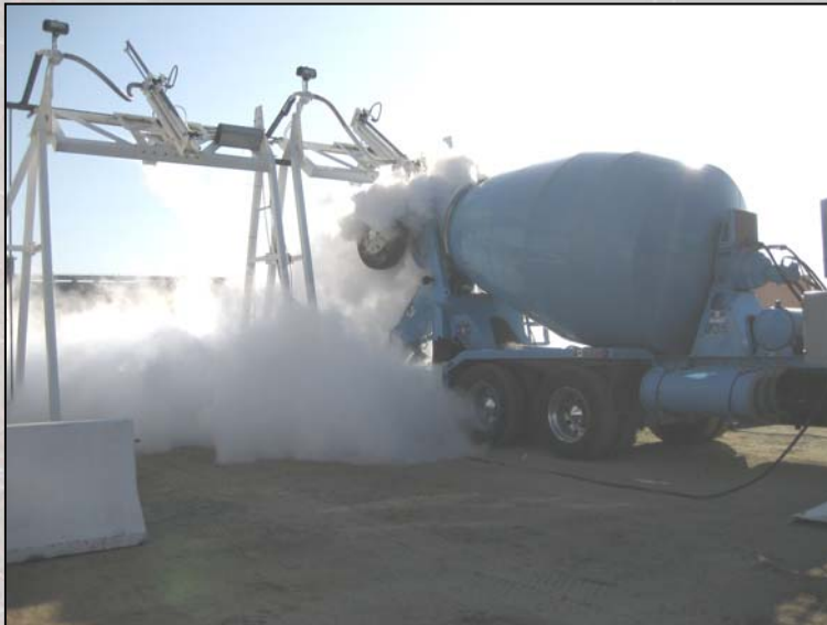
Liquid Nitrogen Injection
