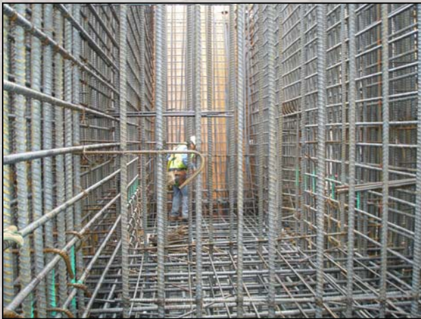
Diaphragm Rebar
