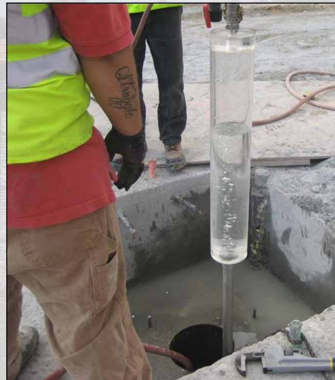
Water Pressure Test
