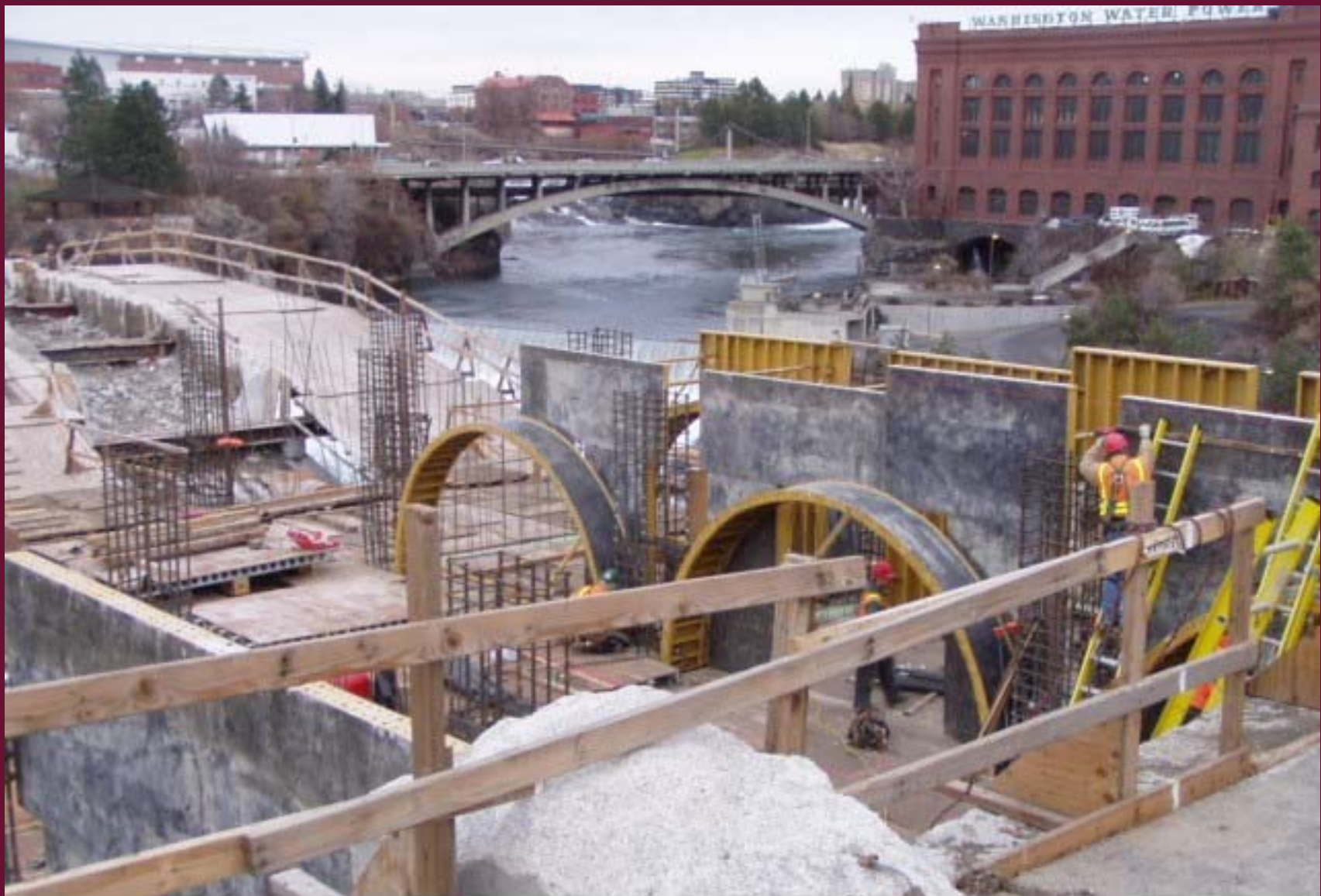
Setting wood grade strip on Steel Form Dec./04
