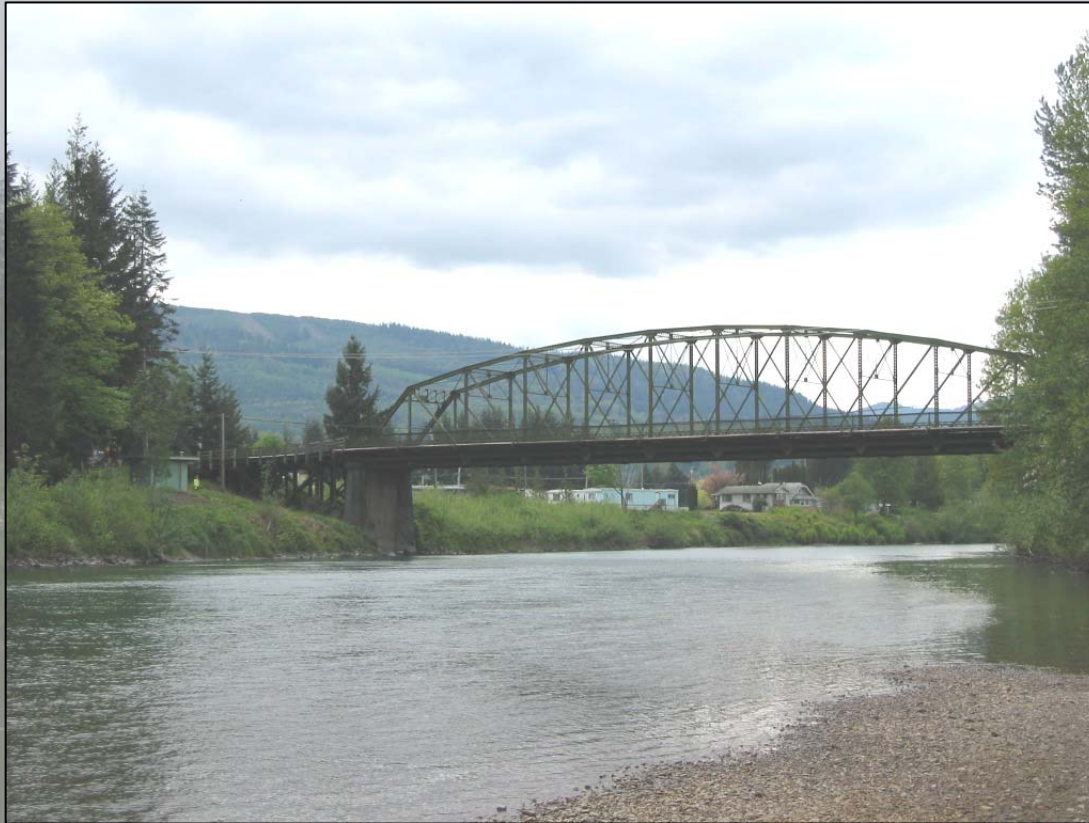
Meadowbrook Bridge looking West- Down stream
