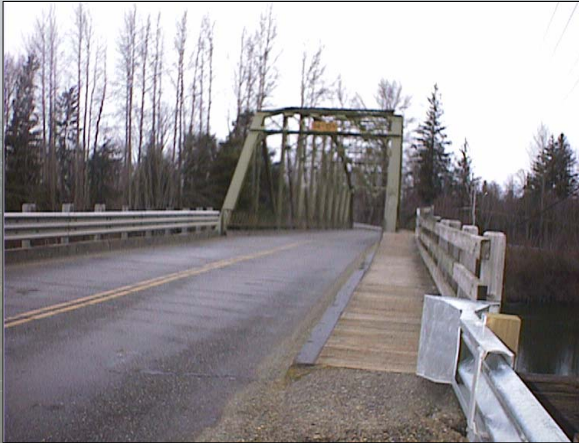
Meadowbrook Bridge looking North
