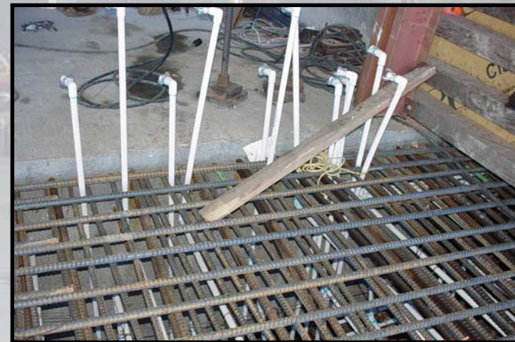
Post Cooling with Water Running through PVC Tubing
