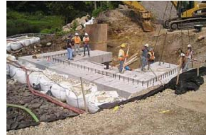
Figure 3.2.1.2-2 Completed footing.
