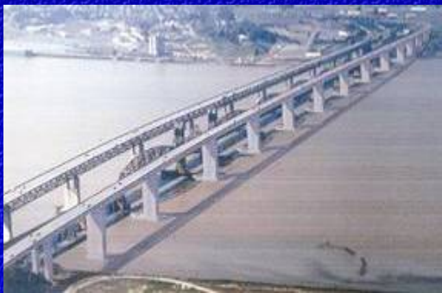
New Benicia-Martinez Bridge (2007) Also LWC Deck on Ex. Truss (1962)
