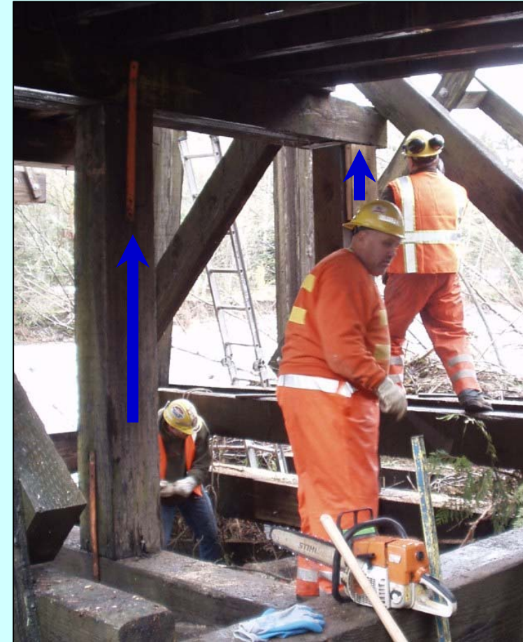
BARING BRIDGE - Loss of two Approach Support Posts below West Tower
