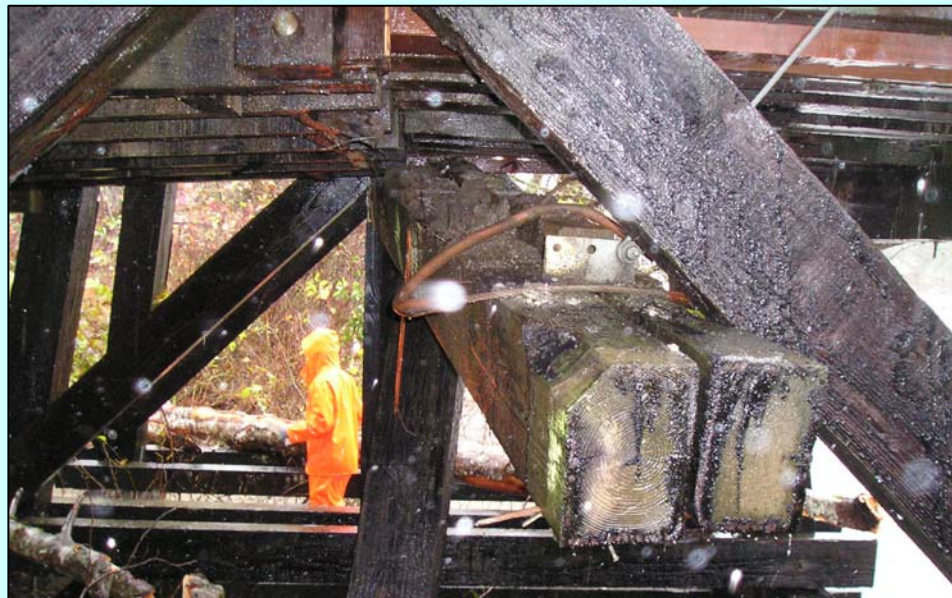
BARING BRIDGE - Loss of two Approach Support Posts below West Tower
