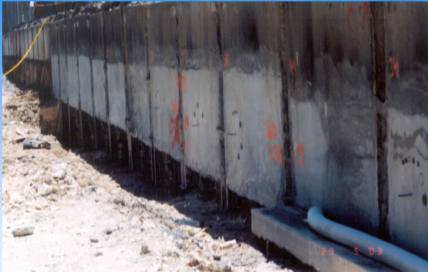
FIG. 2 TIED-BACK SOLDIER PILE WALL SHOWING CIP CONCRETE LAGGING
