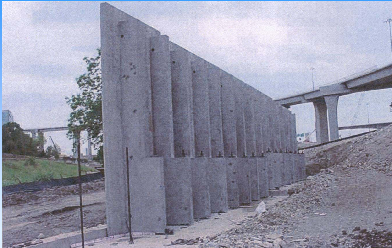
FIG. 7 ERECTED DOUBLE-T PANELS
