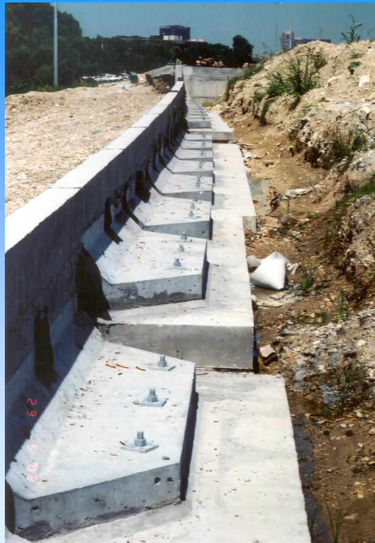
FIG. 4 L-PANELS ON CIP CONCRETE FOOTINGS
