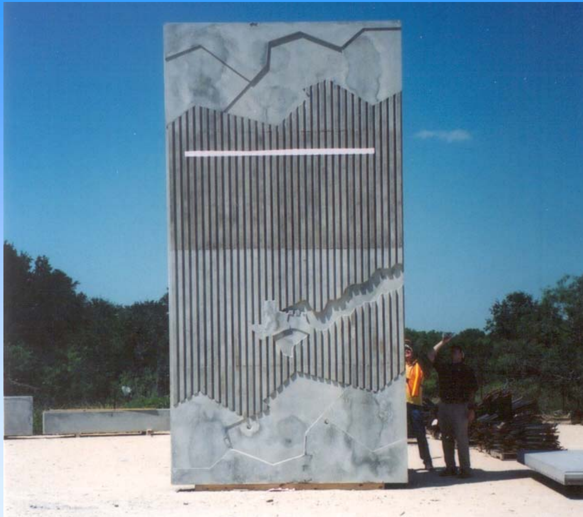
FIG. 3 FULL-HEIGHT FASCIA PANEL FOR SOLDIER PILE WALLS
