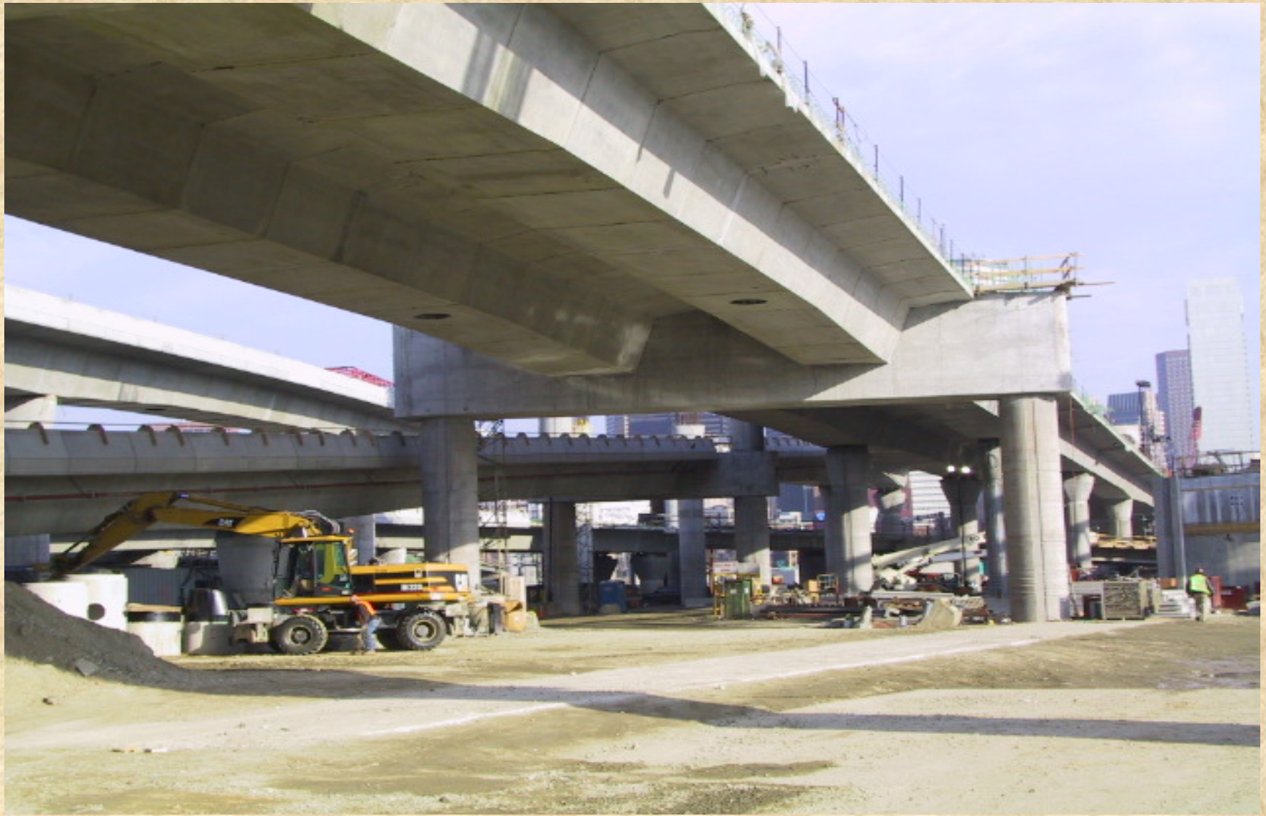
STRADDLE BENT – AFTER ERECTION IS COMPLETED
