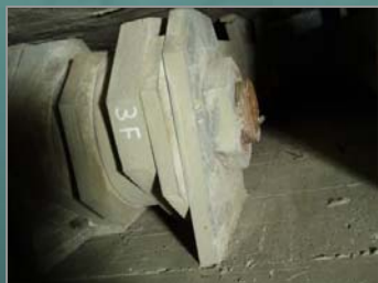
Pin and Hanger Assemblies
