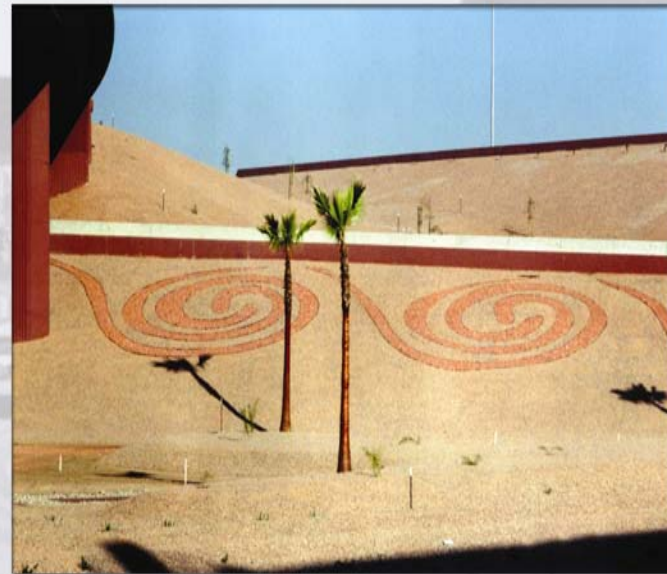
Pima Freeway/ Red Mountain Interchange
