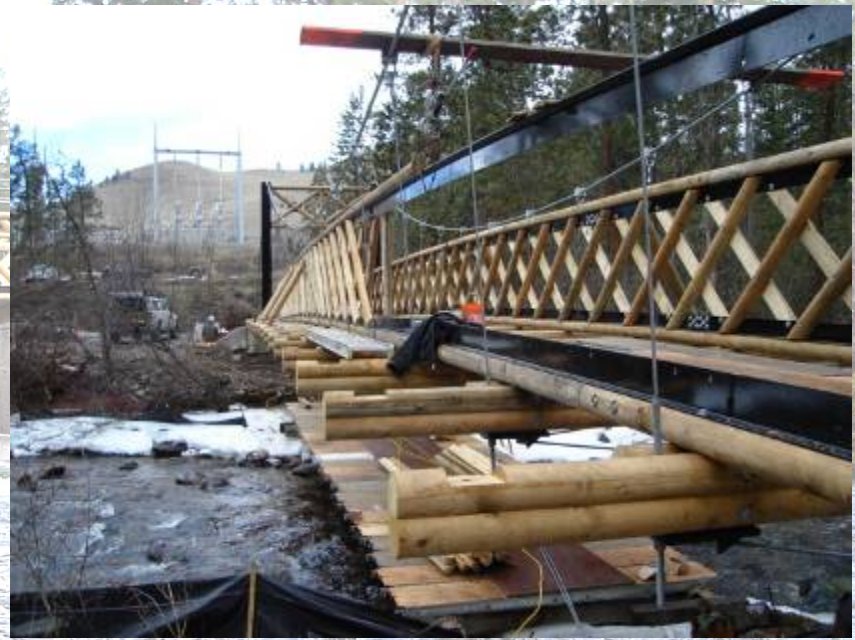
Floor-beams, Braces, and Stiffening Trusses
