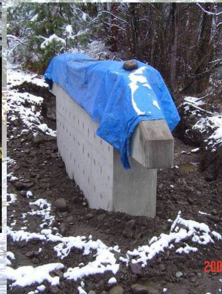
Pier Tower Footings
