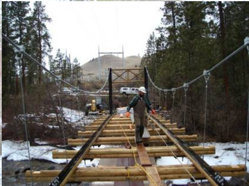
Floor-beams, Braces, and Stiffening Trusses
