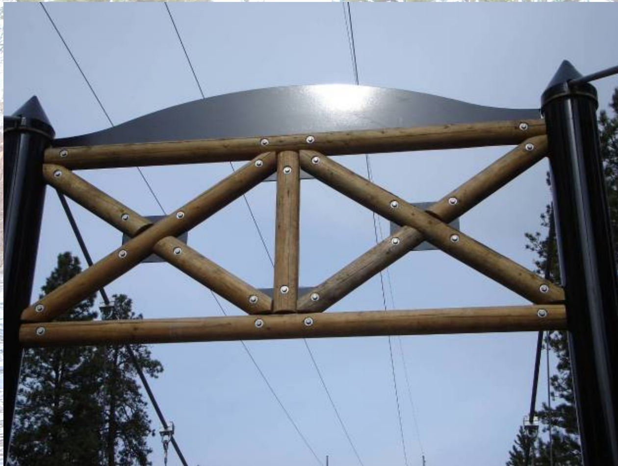
Steel Plates and Cones Installed on Towers as Climbing Deterrent
