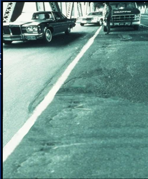
1960 Asphalt Covered Deck
