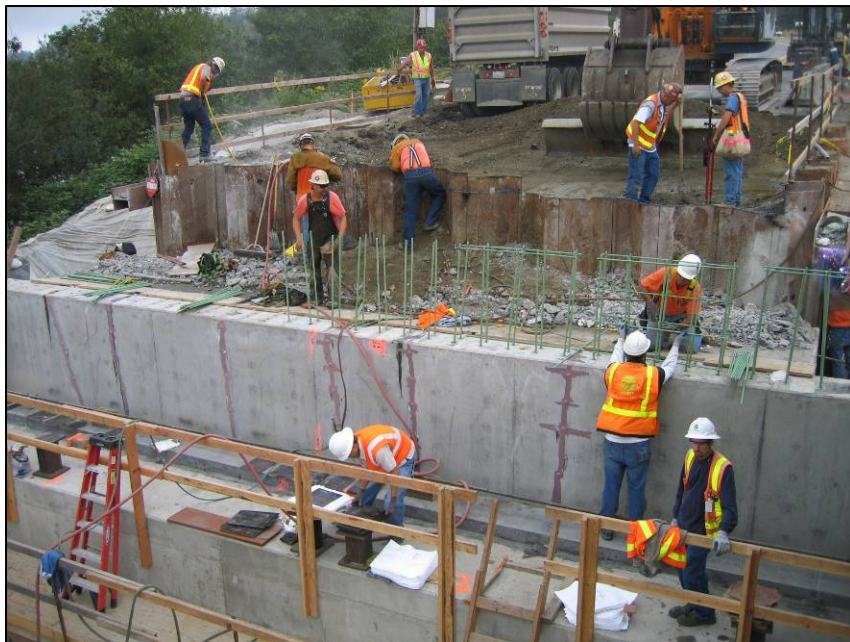
Cast-in-Place Endwall
