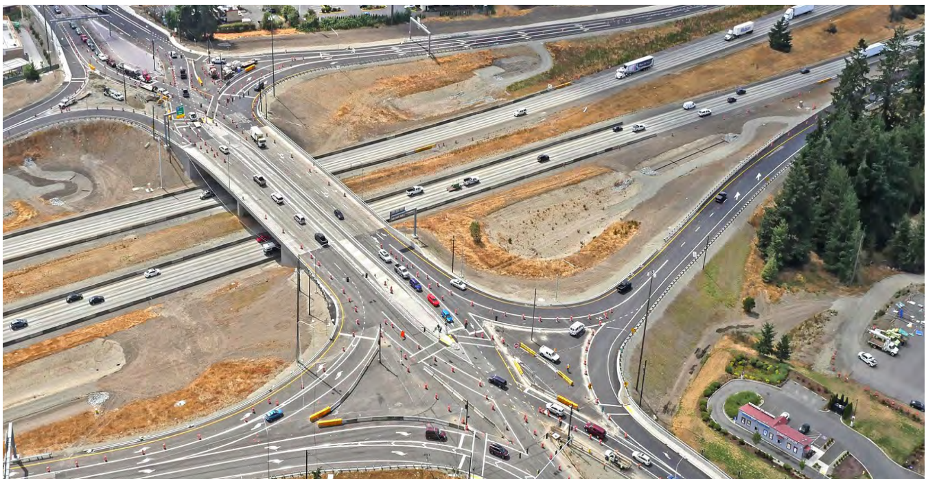
The SR 510 diverging diamond in Lacey was the first of its kind in Washington and significantly reduced the number of potential conflict points for travelers entering and exiting I-5 from the busy state route.
