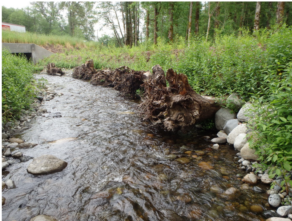
Exhibit 8: Logs and rocks used in restoration.
