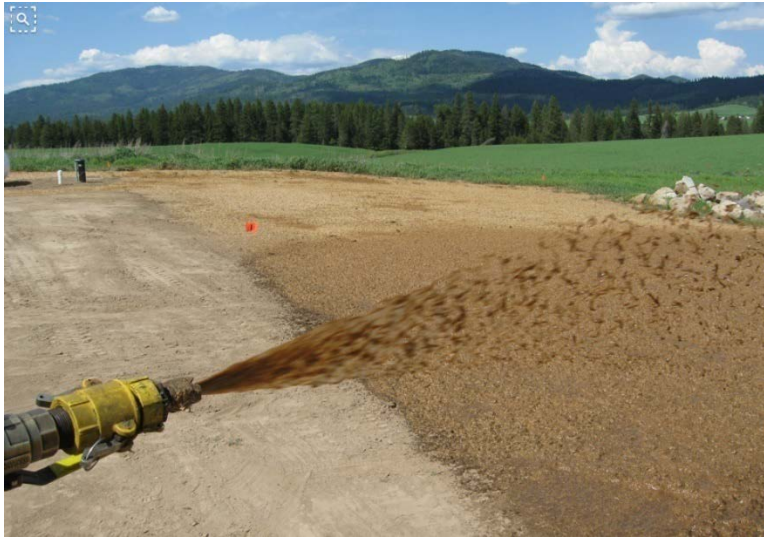
Exhibit 10: Application of hydromulch for erosion control.
