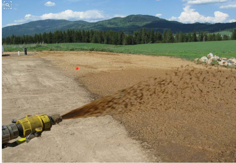
Exhibit 10: Application of hydromulch for erosion control.
