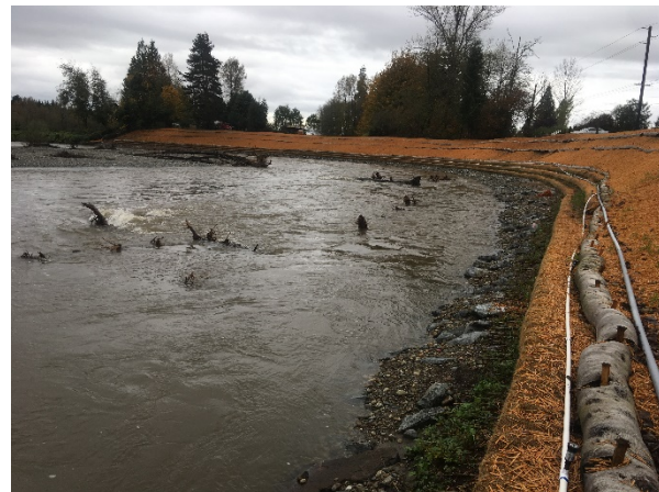
Exhibit 13: SR 92 Pilchuck River Chronic Environmental Deficiency Repair – constructing bank protection and bank protection during first storm.
