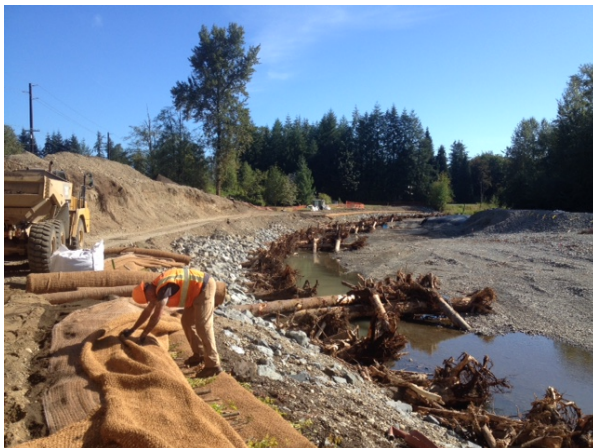
Exhibit 13: SR 92 Pilchuck River Chronic Environmental Deficiency Repair – constructing bank protection and bank protection during first storm.
