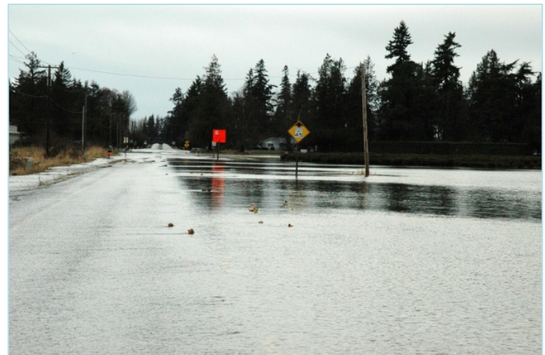
SR 11 during the 2009 Flood Event
