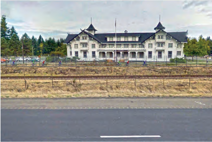
Figure 4.11-4 View at Lewis Army Museum from Southbound I-5 with Proposed Shared Use Path
