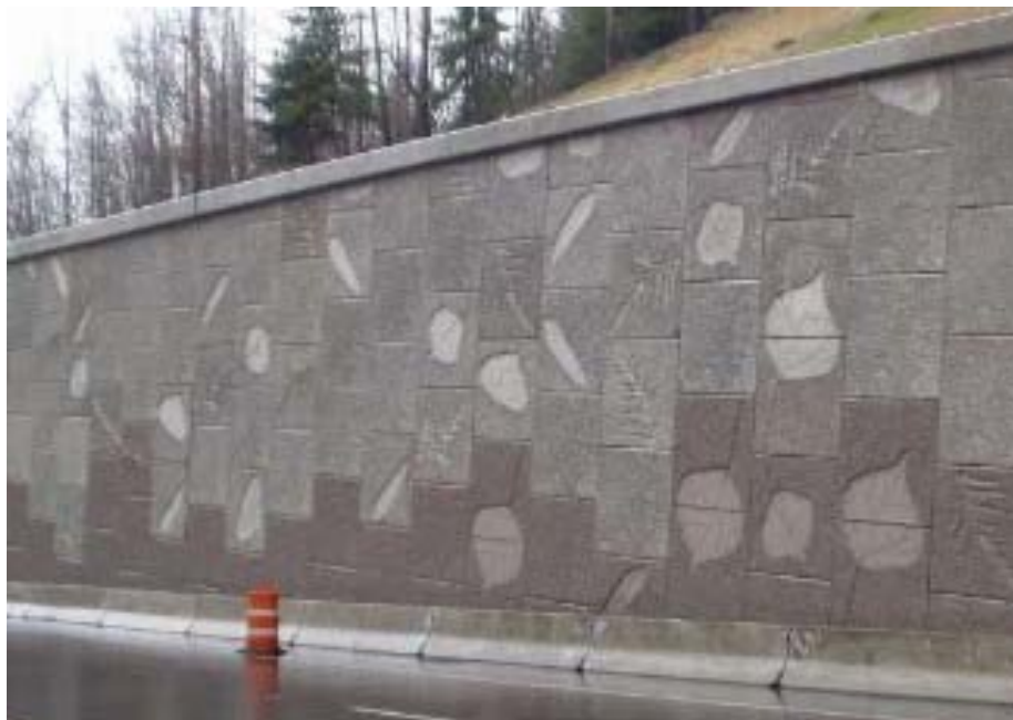
Figure 910.2 Leaf Pattern on retaining wall at I-90 Sunset Interchange
