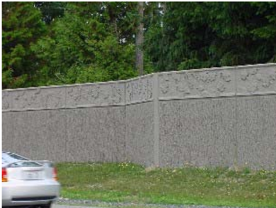
Figure 910.1 Noise wall enhancement in Mill Creek
