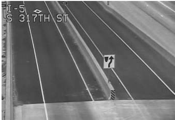
Keep Right sign located at the top of the median barrier separating on- and off-ramps.
