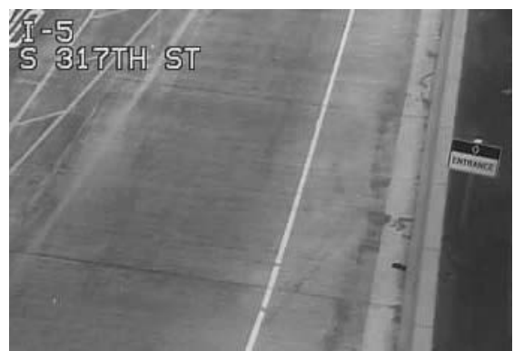
HOV Entrance sign located on the right side at the beginning of each on-ramp.
