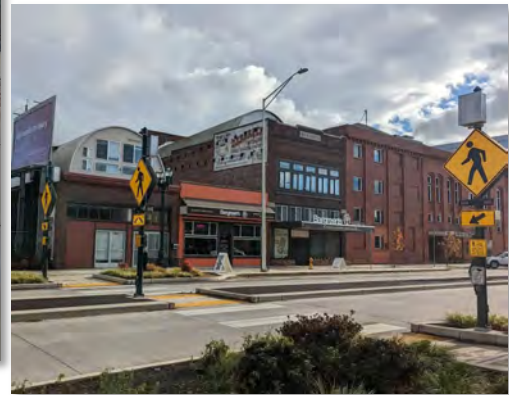
Rectangular rapid flashing beacons
