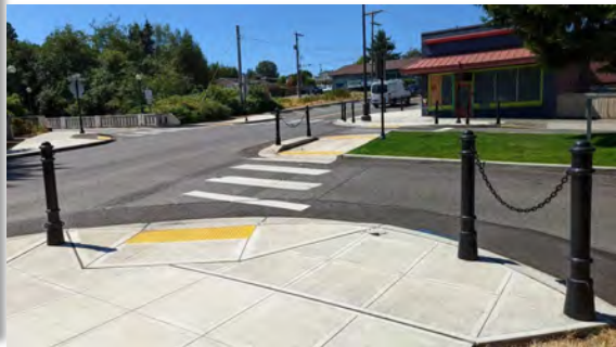
ADA ramps and marked crosswalk
