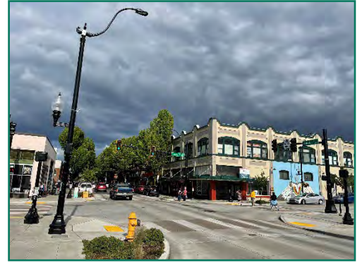
FIGURE 42. TRAFFIC SIGNAL IN OLYMPIA, WA
