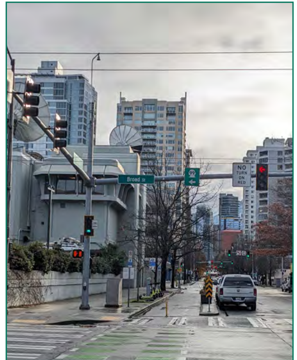
FIGURE 45. PROTECTED-LEFT-TURN SIGNAL IN SEATTLE, WA.
