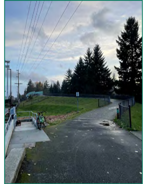
FIGURE 53. PEDESTRIAN/BICYCLIST OVERPASS IN OLYMPIA, WA.
