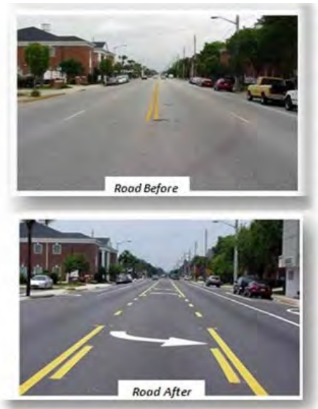
FIGURE 10. ROAD RECONFIGURATION. SOURCE: FHWA.
