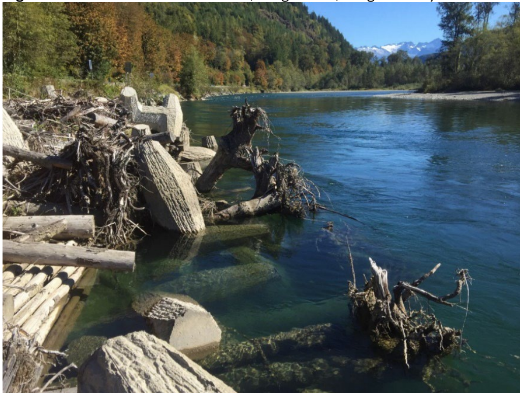
Figure 10A-9 Dolotimber Structures, Skagit River, Skagit County
