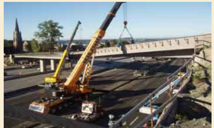
Cranes lift a girder into place for the new Delin Street overpass.
