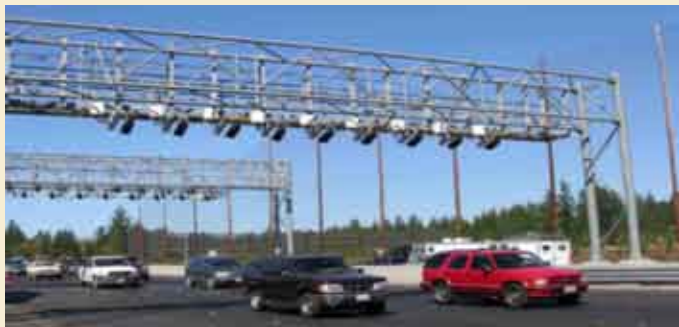
Gantries automatically scan transponders as cars enter the bridge
