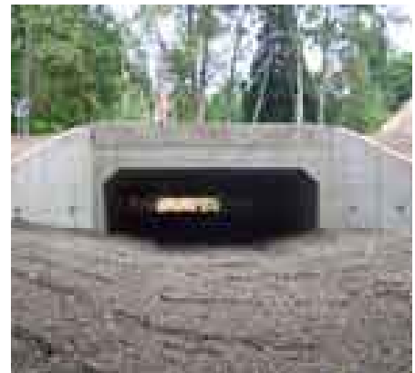
A new concrete culvert will allow fish to pass beneath SR 548 in a more natural streambed
