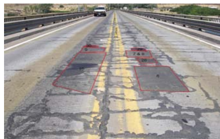
Deteriorated concrete deck to be replaced on U.S. 97 Columbia River Biggs Rapids Bridge.
