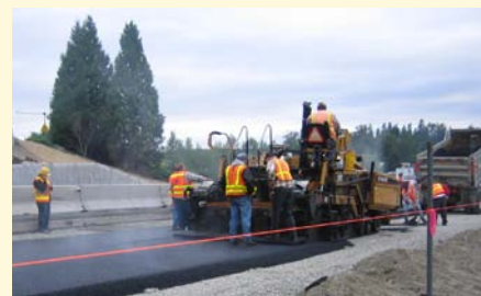
Crews place HMA with an asphalt paving machine on I-405 at Totem Lake.
