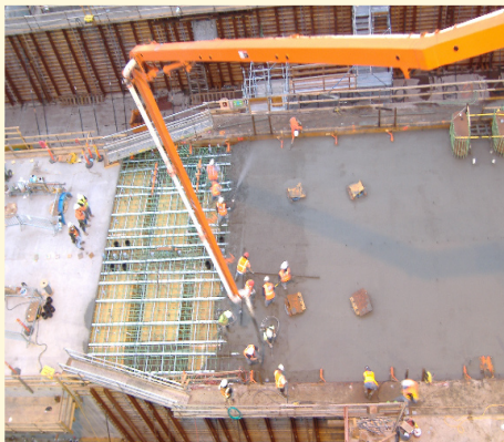
K-G crews smooth concrete during the final top deck pour for Pontoon PA.
