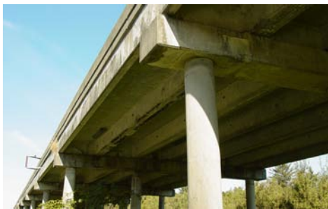
Concrete girders to be repaired under U.S. 2 Ebey Island Viaduct.
