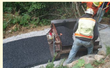
Workers place HMA with a spreader box to create a paved walkway at the Iron Goat Interpretive Center.
