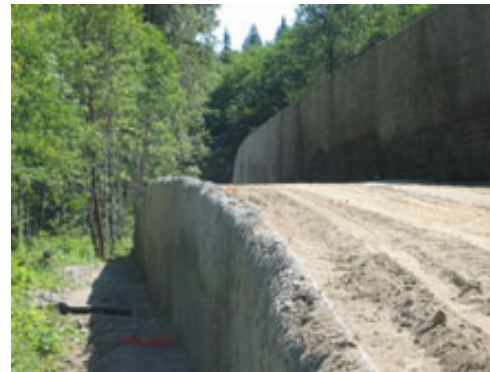
On SR 530 in Darrington, crews built a retaining wall to prevent future mudslides.
