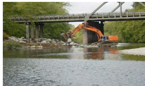
Scour Mitigation Project at the U.S. 101 Humptulips Bridge.
