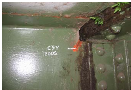
Fatigue cracking on a steel stringer connection on I-5 East Fork Lewis River Bridge.
