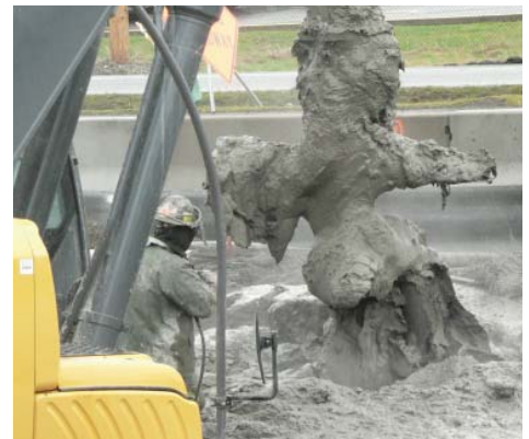
Dwarfed by a massive drill bit and crane, a worker monitors this construction work to ensure safety and efficient production. This work will strengthen and support bridge piers for a new northbound I-5 bridge over the Puyallup River.
