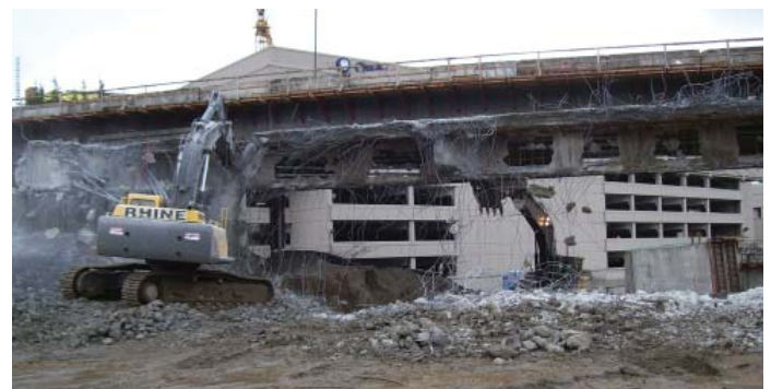
Crews use large crunchers to take down the old NE 12th Street Bridge over I-405. Six to eight inches of sand has been laid on the I-405 roadbed to protect it from debris.
