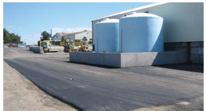
The walled secondary containment unit for salts ensures that any spillage is prevented from reaching the pavement in runoff.
