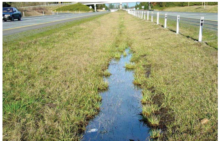
Vegetated filter strip designed to treat highway runoff in the median.
