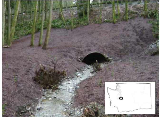
This project improved streambeds and installed new culverts under SR 305 in Kitsap County to remove restrictions to fish passage.
