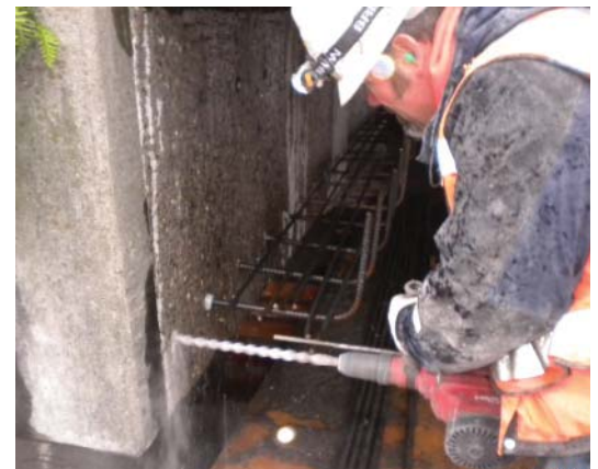
Crews performed seismic retrofits on I-5 bridges in Snohomish County to mitigate earthquake risks.
