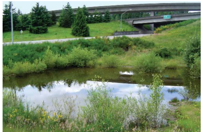
Stormwater infiltration pond near roadway.
