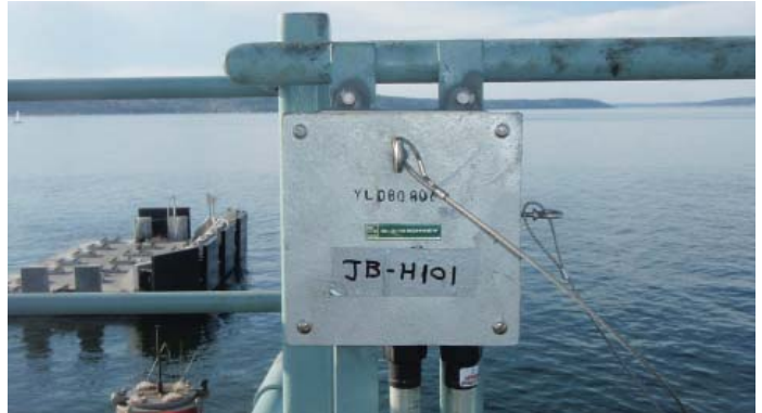
Mukilteo ferry terminal preservation, March, 2011 – A new junction box mounted on new headframe hand rails. The new floating dolphin can be seen in the background. This view looks toward Whidbey Island.
