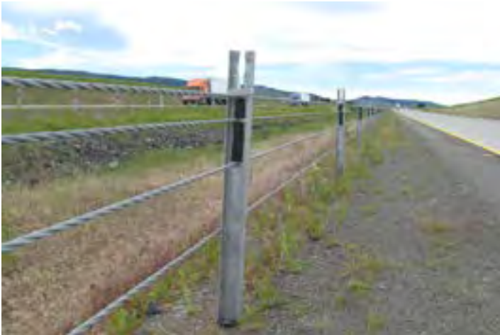
A four-strand, high-tension cable median barrier system.
