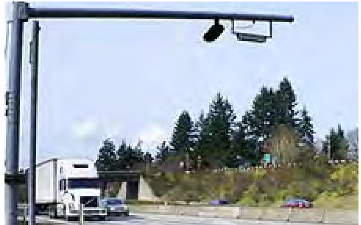
An Automated License Plate Recognition device and transponder reader (on top of the pole, right) relay information to commercial vehicle enforcement officers about a truck as it approaches a weigh station.
