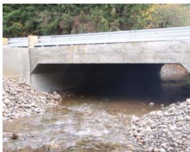
A 5-foot culvert was a barrier on the South Branch of Big Creek on SR 101. It was replaced with this new 21-foot culvert, improving access to fish habitat.
