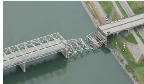
Aerial view of the I-5 Skagit River Bridge near Mount Vernon, which collapsed on May 23, 2013 after a truck collided with the steel framework.
