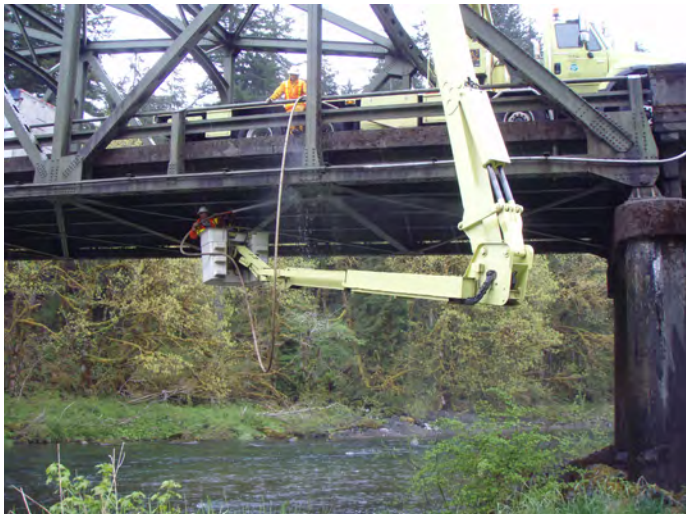
Crews wash a bridge over the Sol Duc River on the Olympic Peninsula. Programmatic permits with Fish and Wildlife allow WSDOT to complete bridge washing without filing for separate permits for each bridge.
