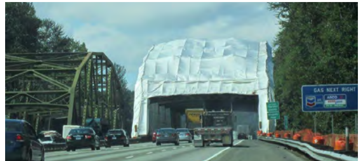
A containment system covering the Southbound Interstate 5 Nisqually River Bridge will keep old paint and paint removal material from entering the environment as the bridge is repainted.
