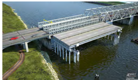
Conceptual design of the finished replacement span before it is installed. Image is used with permission from Max J. Kuney Construction and Parsons Brinckerhoff.
