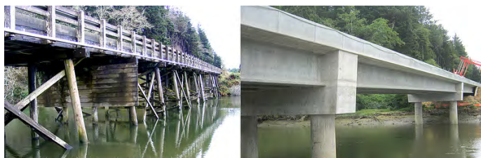
Before and after: Replacement of the structurally deficient and functionally obsolete 1936 U.S. 101 Bone River Bridge. The replacement bridge is a concrete structure built to withstand flooding and major earthquakes.
