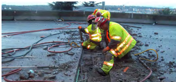
Replacement of an expansion joint, a common bridge repair, on Interstate 5 in Seattle near Beacon Hill in April 2013.
